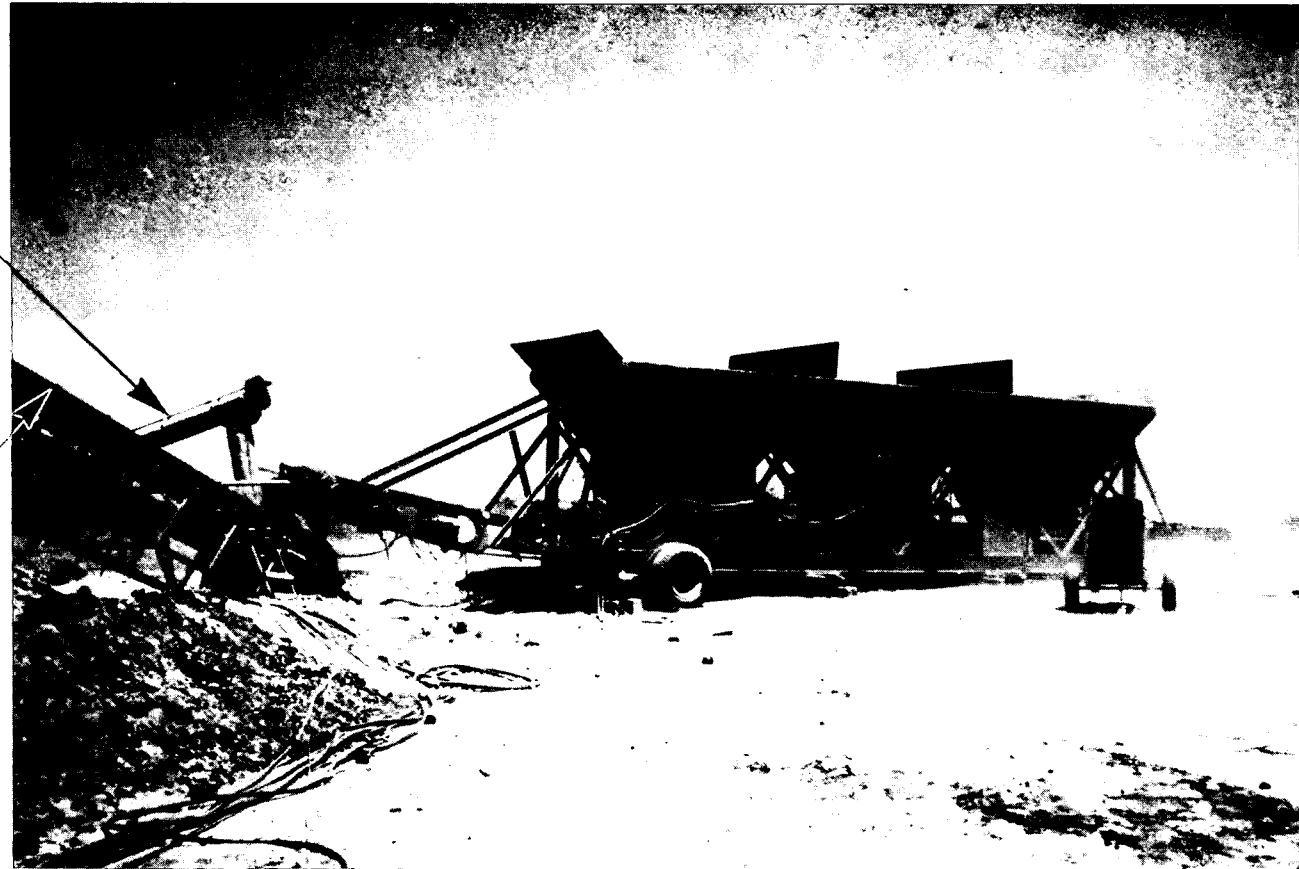
PLATE 1 THREE-BIN COLD-AGGREGATE PROPORTIONER UNIT AND FILLER ADDITION POINT SAFFORD, ARIZONA
