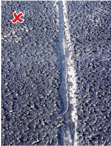
Figure 2.9 Overfilled saw-cut
