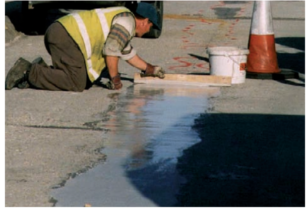
Figure 3.4 A large depression in a deck being filled with repair material
