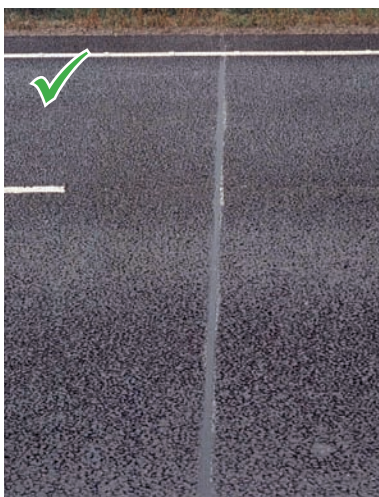
Figure 2.11 Good saw-cut and seal
