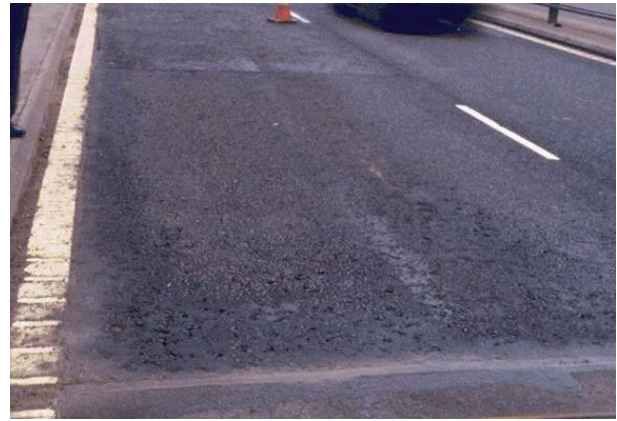
Figure 3.10 Two sections of hot rolled asphalt laid in lane 1 that replaced thin surfacing on high side of expansion joint
