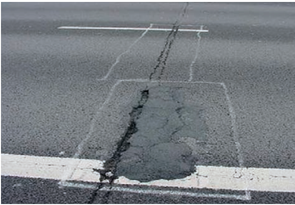
Figure 2.12 Condition of reflection crack prior to treatment
