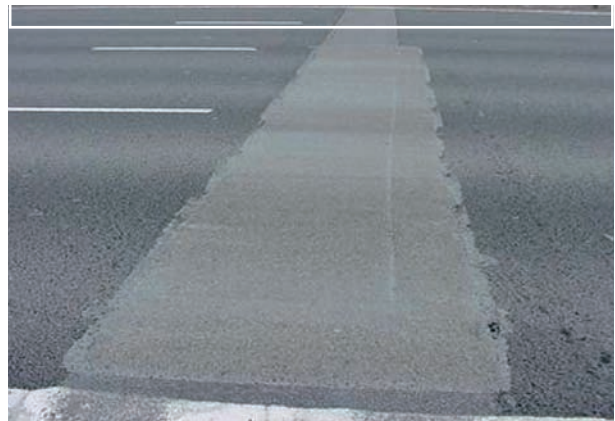
Figure 2.15 Typical patch repair
