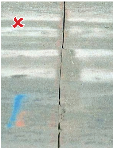
Figure 2.7 Spalling of the saw-cut, no strike plate used
