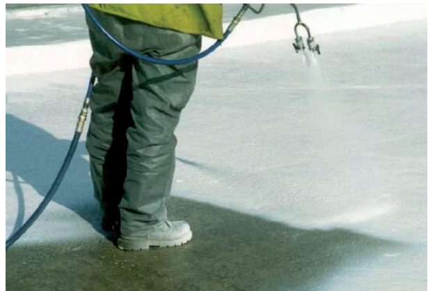
Figure 3.13 Applying a waterproofing membrane
