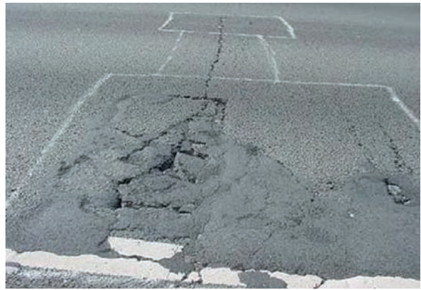
Figure 2.13 Condition of reflection crack prior to treatment
