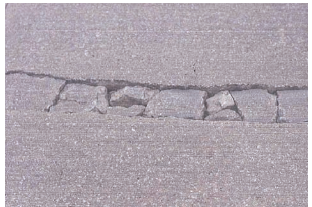
Figure 2.18 Example of major crack defect: A “punchdown”
