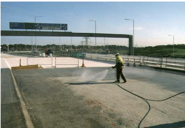
Figure 3.12 Priming a bridge deck
