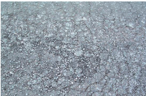
Figure 3.7 Extensive break-up of thin surfacing where high hydrostatic pressures were generated in the saturated surfacing
