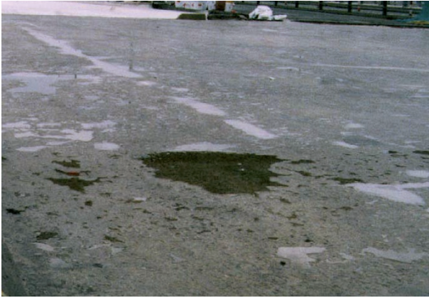
Figure 3.3 A large depression in a primed deck where water has ponded (before it was filled with repair material)
