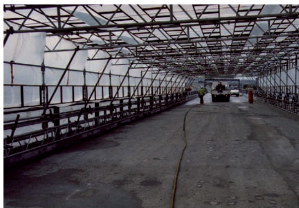
Figure 3.14 A bridge deck tented to enable installation of the waterproofing system in adverse weather
