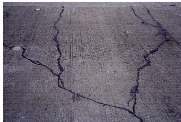
Figure 2.16 Example of a bifurcated crack
