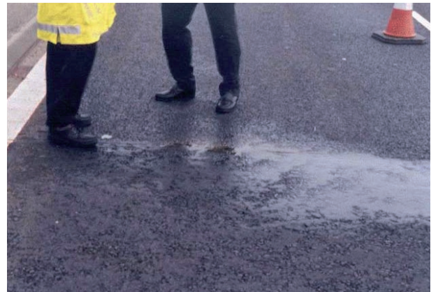
Figure 3.11 Close-up of far end of second section of hot rolled asphalt shown in Figure 3.10 where sub-surface water is coming out of the thin surfacing
