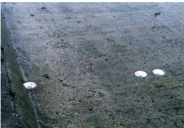
Figure 3.5 Through-deck drains at a location on a bridge that is not free draining
