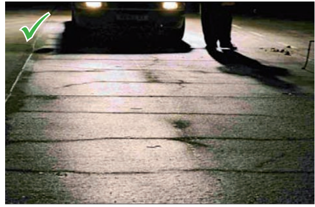
Figure 2.2 Example showing good transverse crack pattern
