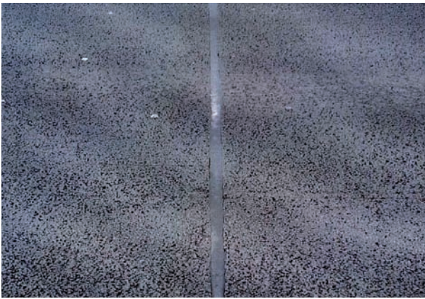
Figure 2.19 Sealed expansion joint
