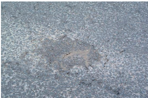
Figure 3.6 Water and fines forced out of a cracked thin surfacing by heavy goods vehicles on a deck with no through-deck drains
