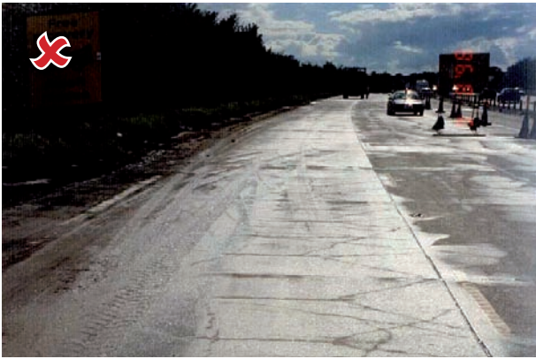
Figure 2.1 Example showing excessive longitudinal cracking
