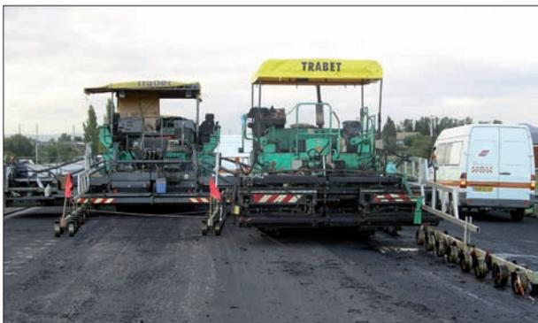
the number of layers not only reduces the number of horizontal interfaces but also leads to thicker layers. The thickness should not exceed that which can be adequately compacted by the plant available, but thicker layers should avoid any problems with thin layer brittleness. Excessively thin layers, in particular binder course, may result in un-designed permeable pavements.
