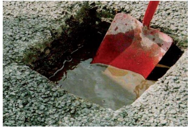
whenever the surrounding material is damp, which will depend on the water table as well as whether there has been any precipitation. If the drains at the side are not maintained and water is held in them, that water is available to enter the side of the pavement for extended periods. Water at the sides and bottom of a pavement can be at higher pressures, encouraging its entry into available voids and any unbonded joints.
