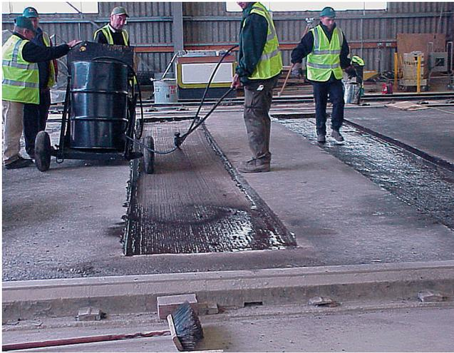
**Figure 6.3** Bitumen emulsion tack coat being applied to the trenches
