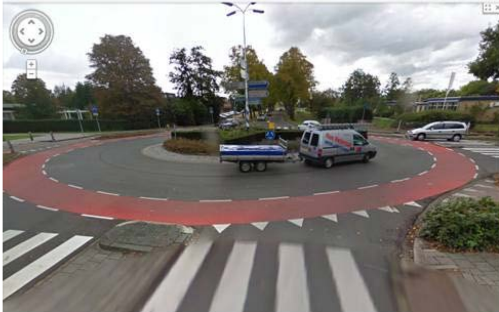
Figure 8: Roundabout in the Netherlands with marked cycle lane
