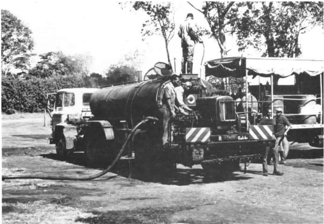
Plate 1 Preparing blended binder (80/100pen and diesel fuel loaded simultaneously)
