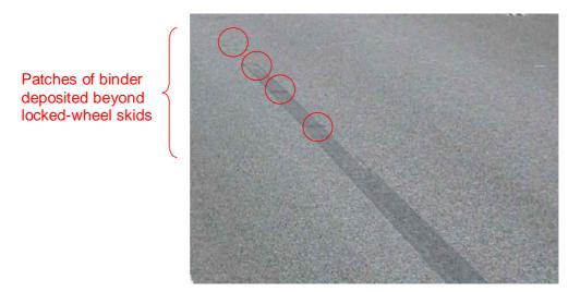
Figure 9.2: patches of transferred binder visible at the end of a skid mark
