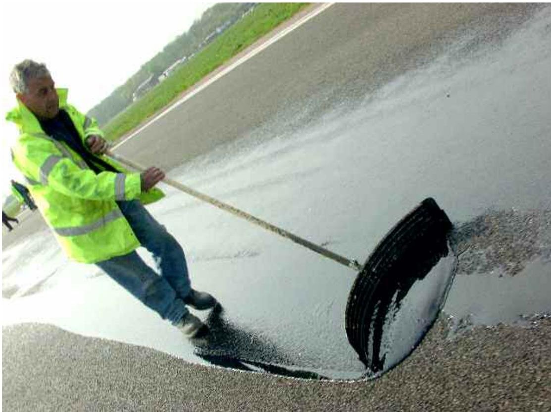
**Figure A2 Waste Engine Oil being spread on Asphalt**
