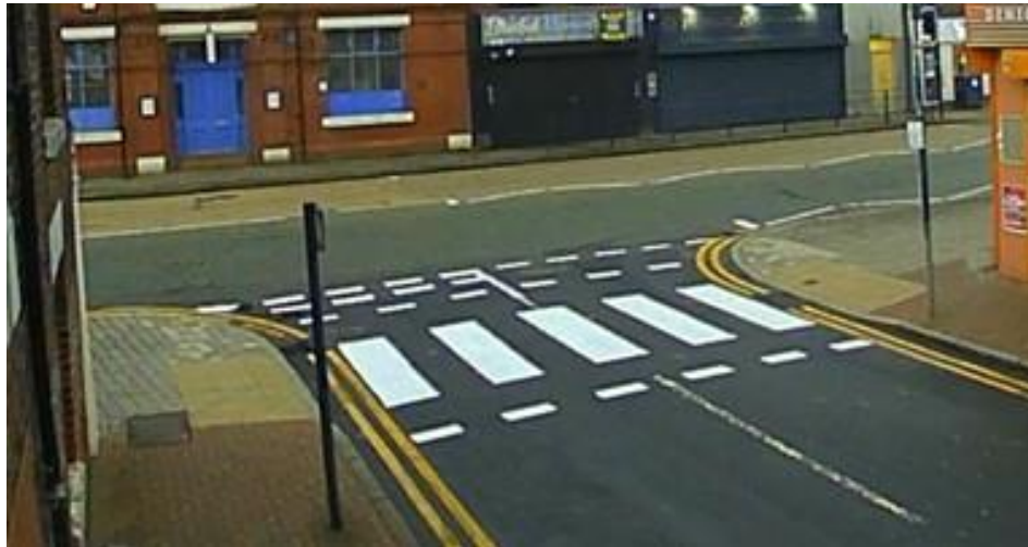
Figure 1: Example of a non-prescribed zebra crossing at one of the trial sites (from video)
