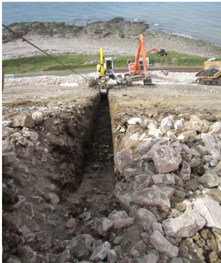
Figure 3.1: Construction of a Counterfort Drain on a steep slope (26°) above a live railway line on the Cumbrian Coast Railway. The counterfort is being constructed using a Menzi Muck slope climbing excavator with a winch line (image the authors)
