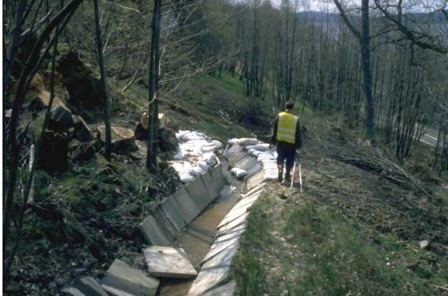
Figure 3.13: A particularly poor example of drainage constructed as part of a Regrade (image the authors)
