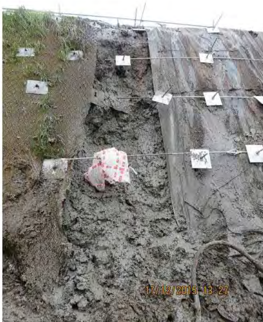
Figure 1: Extract of construction phase pre-nailing/facing failure, Soil Nail Slope 1 Plate 27 (image) taken from A1L2B Geotechnical Feedback Report.
