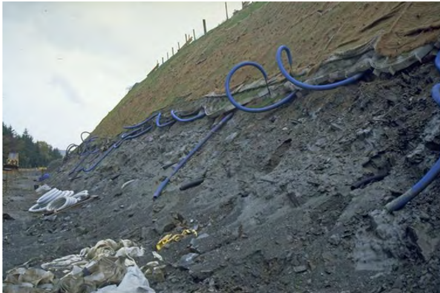
Figure 3.17: Construction of the A7 Colterscleuch Soil Nail slope in 1994 (image the authors)
