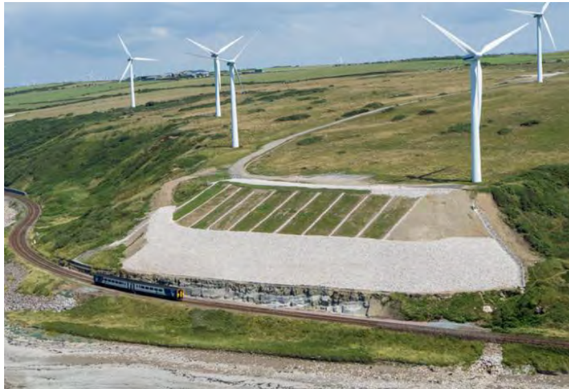
Figure 3.4: Regraded slope on the Cumbrian Coast Railway with Counterfort Drains. The upper slope above the rock fill blanket is clayey till and the area covered by the rock fill blanket is glacial sand (believed to be an esker). The counterforts also have slope (herring bone) drains to pick up localised water, they are generally concealed by the rock blanket. The top of one such slope drain can be seen on the fourth counterfort from the left side, as shown in Figure 3.3. This highlights the need for detailed as built records to aid with future inspections, analysis and maintenance (image J Murphy and Sons Ltd.)
