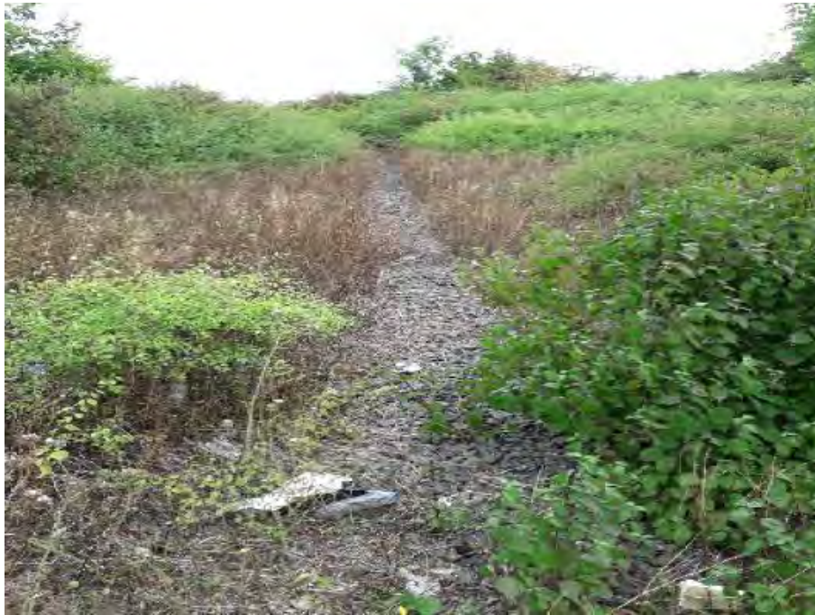
Figure 3.6: Build-up of vegetation within the Counterfort Drain leading to a reduction in functionality along the A14: M1 J19 to A14 J1 (from Kier, 2019)
