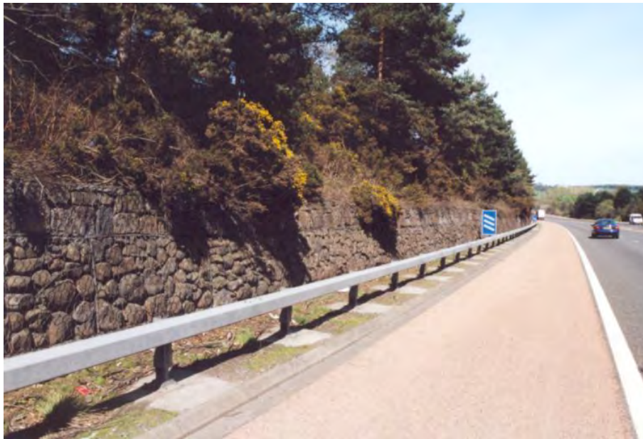
Figure 3.11: Gabion Wall faced with waste building stone, M876 Junction 1 to Junction 2 (from Winter & Anderson, 2002)
