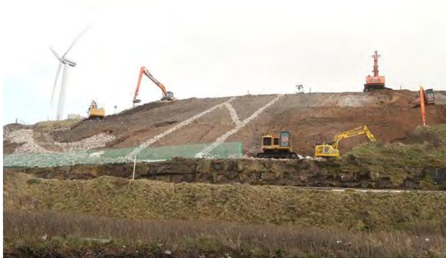
Figure 3.3: Regraded slope on the Cumbrian Coast Railway with Counterfort Drains. The upper slope is clayey till and the lower slope is glacial sand believed to be an esker. The counterforts also have slope (herring bone) drains to pick up localised water. The slope drain on the second counterfort from the left is just evident on the completed slope in Figure 3.4 (image the authors)
