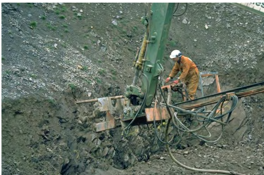
Figure 3.18: Construction of the A74 (M74 Junction 14 to 15) Tinny Bank soil nail trial in 1994/5 (lack of guarding on the drill rig due to date) (image the authors)
