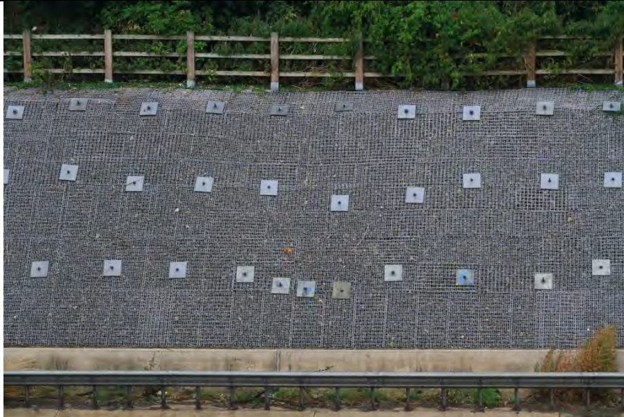
Figure 3: Photograph of SNS2 showing nail placement (old and replacement)
