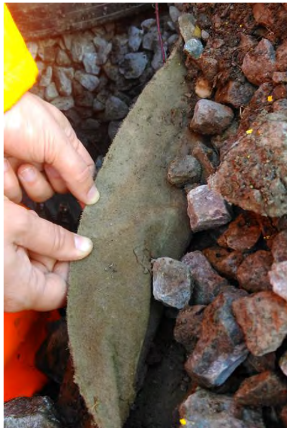
Figure 3.5: Drain with a smeared geotextile and contaminated granular drainage aggregate (image the authors)
