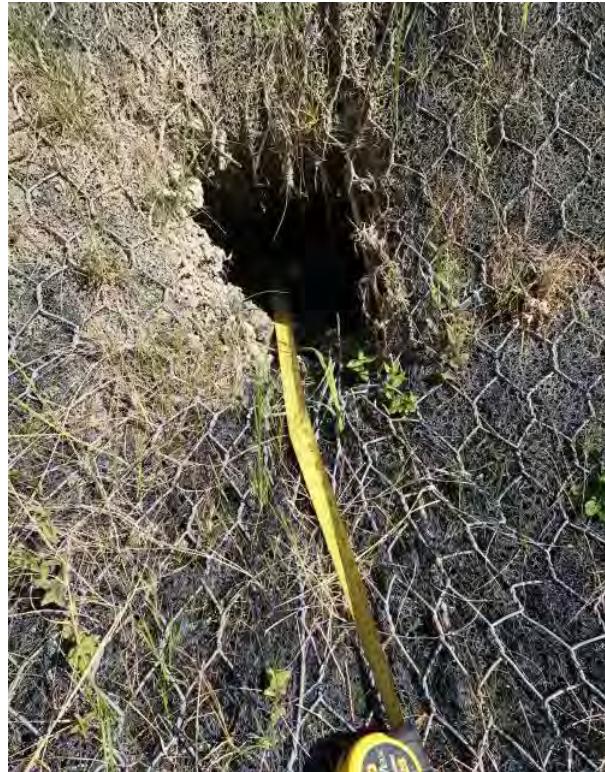
Figure 3.22: Mesh soil nail slope facing where the slope movement forces have caused punching failure of the soil nail mesh facing. The face plate is approximately 600mm back from the facing (image the authors)
