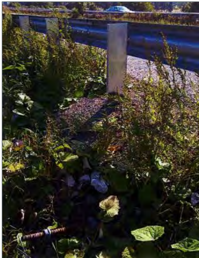
Figure 1. Extract of Damaged Soil Nail Photograph 1 (image) taken from BBMM 2011 Report.
