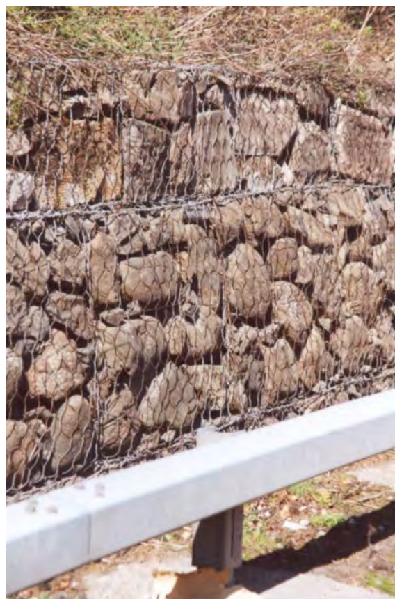
Figure 3.12: Gabion Wall faced with waste building stone, M876 Junction 1 to Junction 2 (image the authors)
