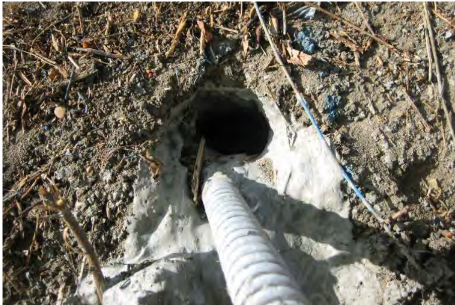
Figure 3.21: Soil nail lying on the base of the borehole due to failure to use centralisers. This reduces the grout cover for corrosion protection and potentially reduces the bond strength (image the authors)
