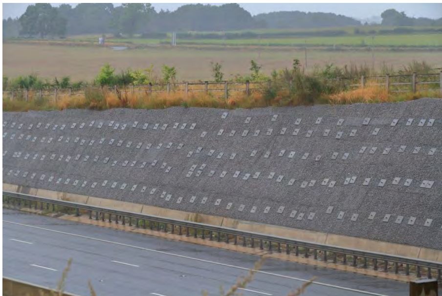
Figure 4: Photograph of SNS1 showing nail placement (old and replacement)
