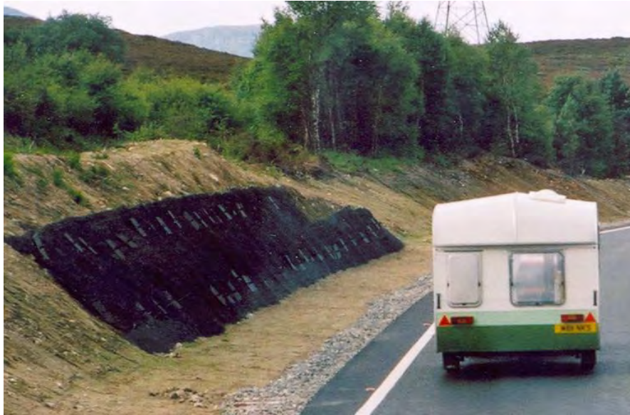
Figure 3.20: Example of a low-height Soil Nail reinforced slope (image the authors)
