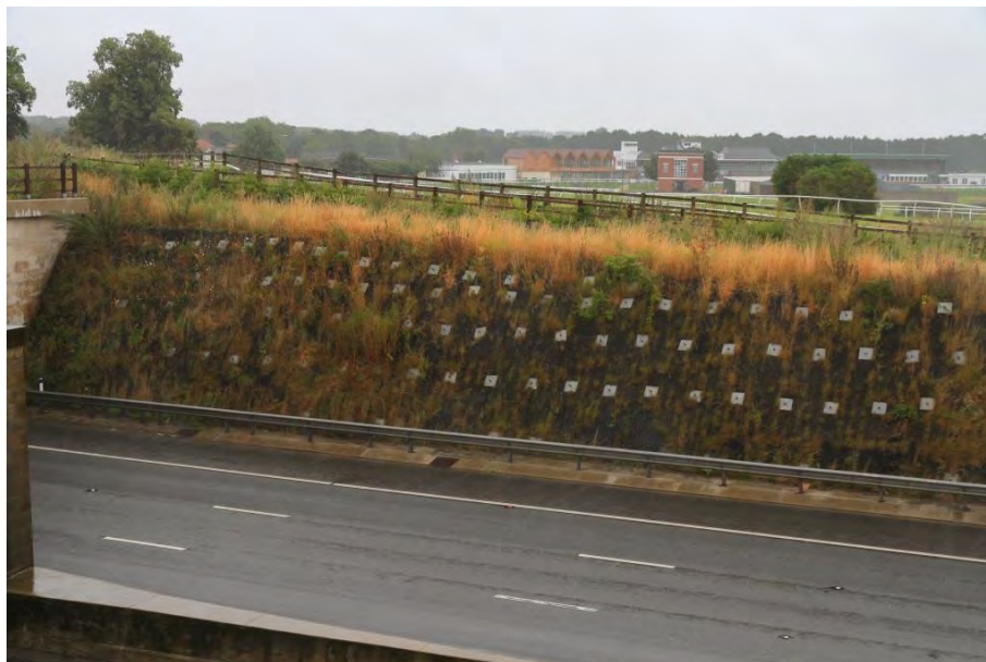
Figure 5: Photograph of SNS3 showing replacement facing product
