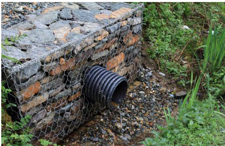
Figure 3.10: Well-constructed gabion basket filled with a stone that has the potential to deteriorate in the environment in which it is placed (image the authors)
