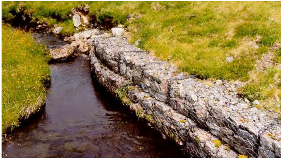
Figure 3.9: Gabion Wall at A835 Loch Dromer showing the embankment being successfully retained by the Gabion Wall, as well as providing bank scour protection, in comparison to the adjacent part of the embankment which is failing (from Winter & Anderson, 2002)
