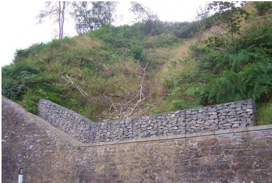
Figure 3.8: Gabion Wall used as a debris trap at B9176 Struie (from Winter et al., 2009)
