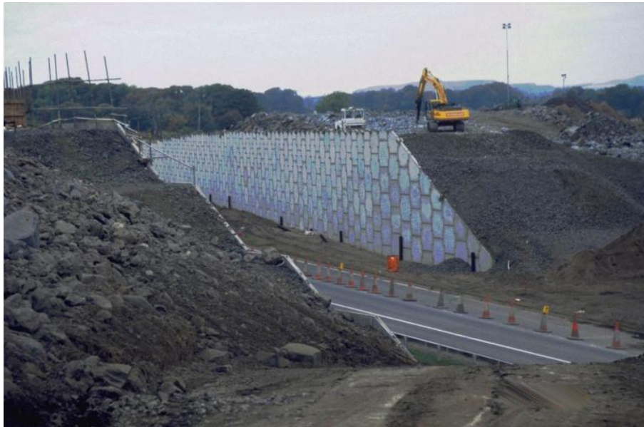
Figure 8: Reinforced soil wall under construction at M8 Junction 2 (Claylands) (from Winter, 1999)
