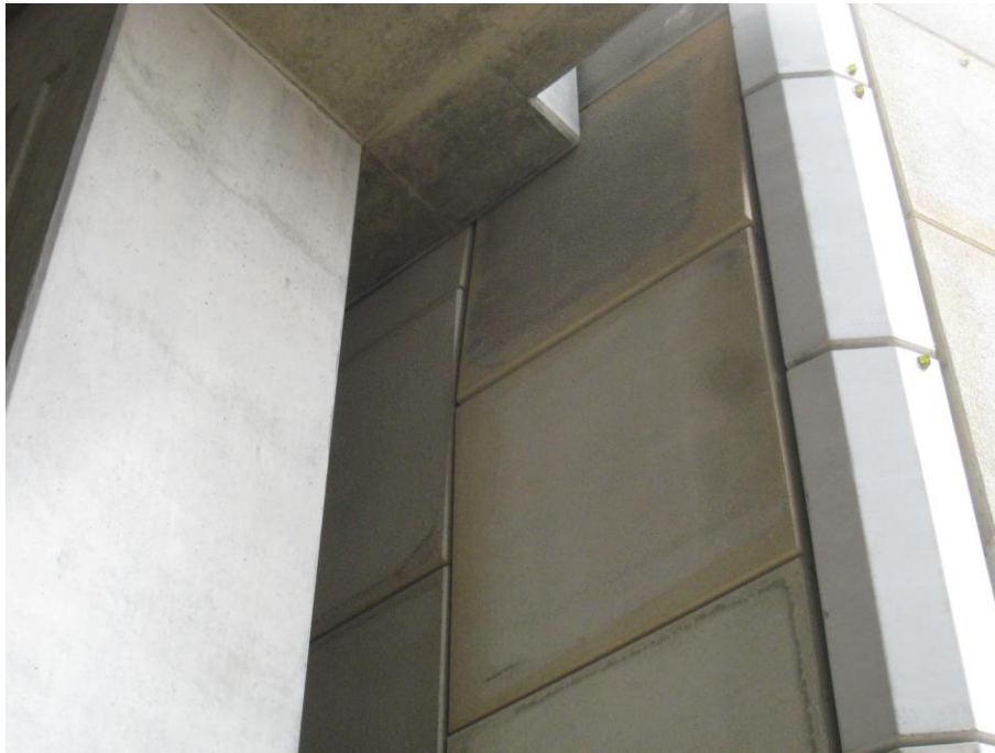
Figure 7: Misalignment of individual facing panels to a polymeric reinforcing; sections of these walls project have been built/rebuilt at least three times (Image National Highways)
