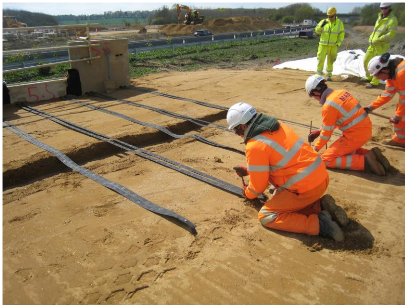
Figure 10: Polymeric reinforcing straps with rigid concrete facing panels showing the trench used to tension the straps along with anchoring of the straps (Image National Highways)
