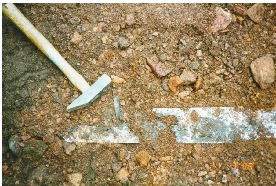
Figure 9: Lindsay Road reinforced soil wall – excavation of ferritic stainless steel reinforcing elements (from Winter et al., 2002)
