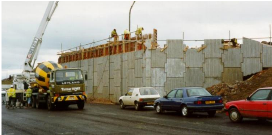
Figure 5: Reinforced soil wall under construction at A96 Brechin Bypass (image the authors)
