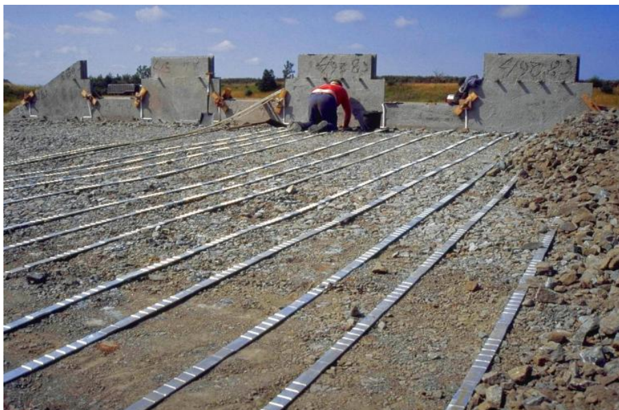
Figure 6: Reinforced soil wall under construction at M8 Junction 2 (Claylands) (from Winter, 1999)
