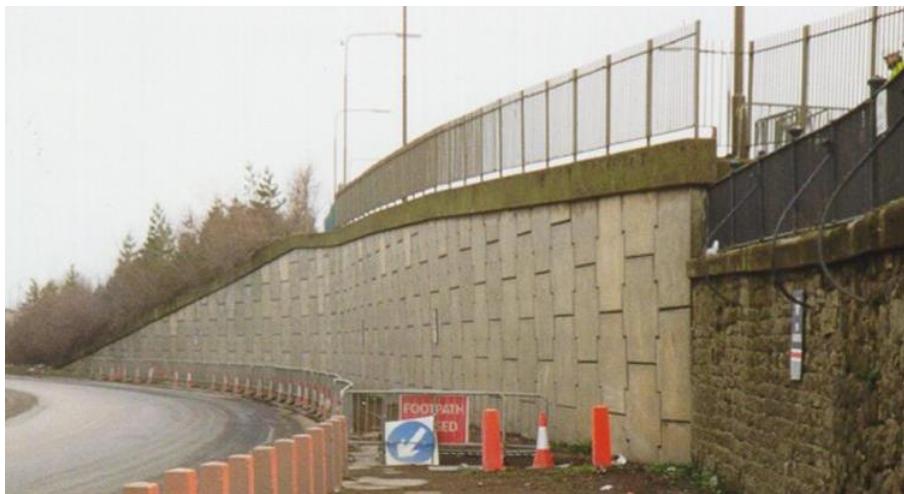
Figure 1: The first reinforced soil wall constructed in the UK at Lindsay Road, Edinburgh (from Winter et al., 2002)
