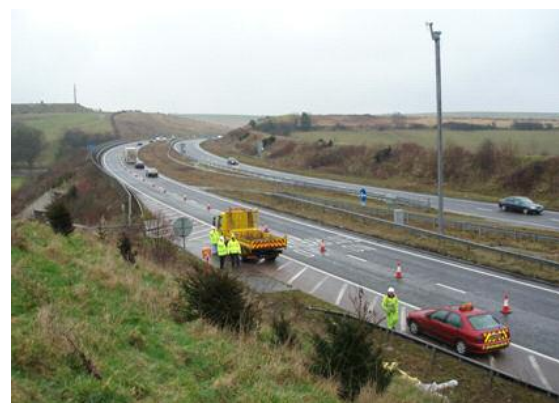
Figure 10: View from the eastern portal of the Southwick Tunnel, looking west.
