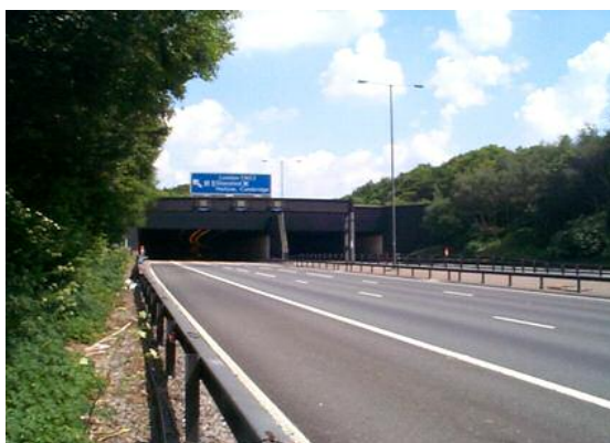
Figure 12: View of the western portal of the Bell Common Tunnel, looking southeast.
