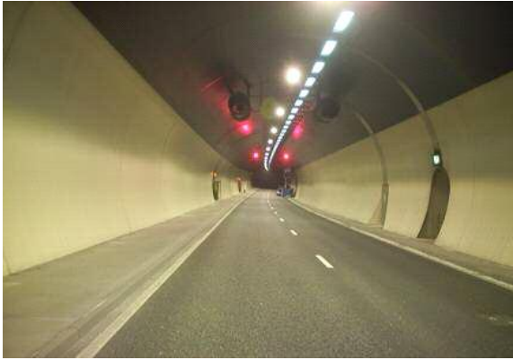
Figure 7: Internal view of the Southwick Tunnel.
