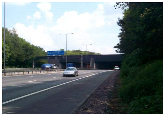
Figure 13: View of the western portal of the Bell Common Tunnel, looking northeast.
