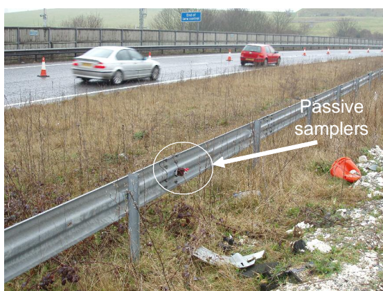
Figure 14: Passive samplers installed on the crash barrier on the edge of the westbound carriage way of the Southwick tunnel eastern portal.
