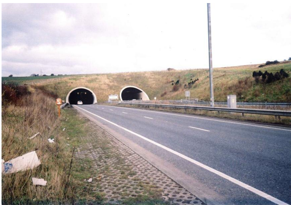
Figure 9: View of the eastern portal cutting of the Southwick Tunnel, looking west.
