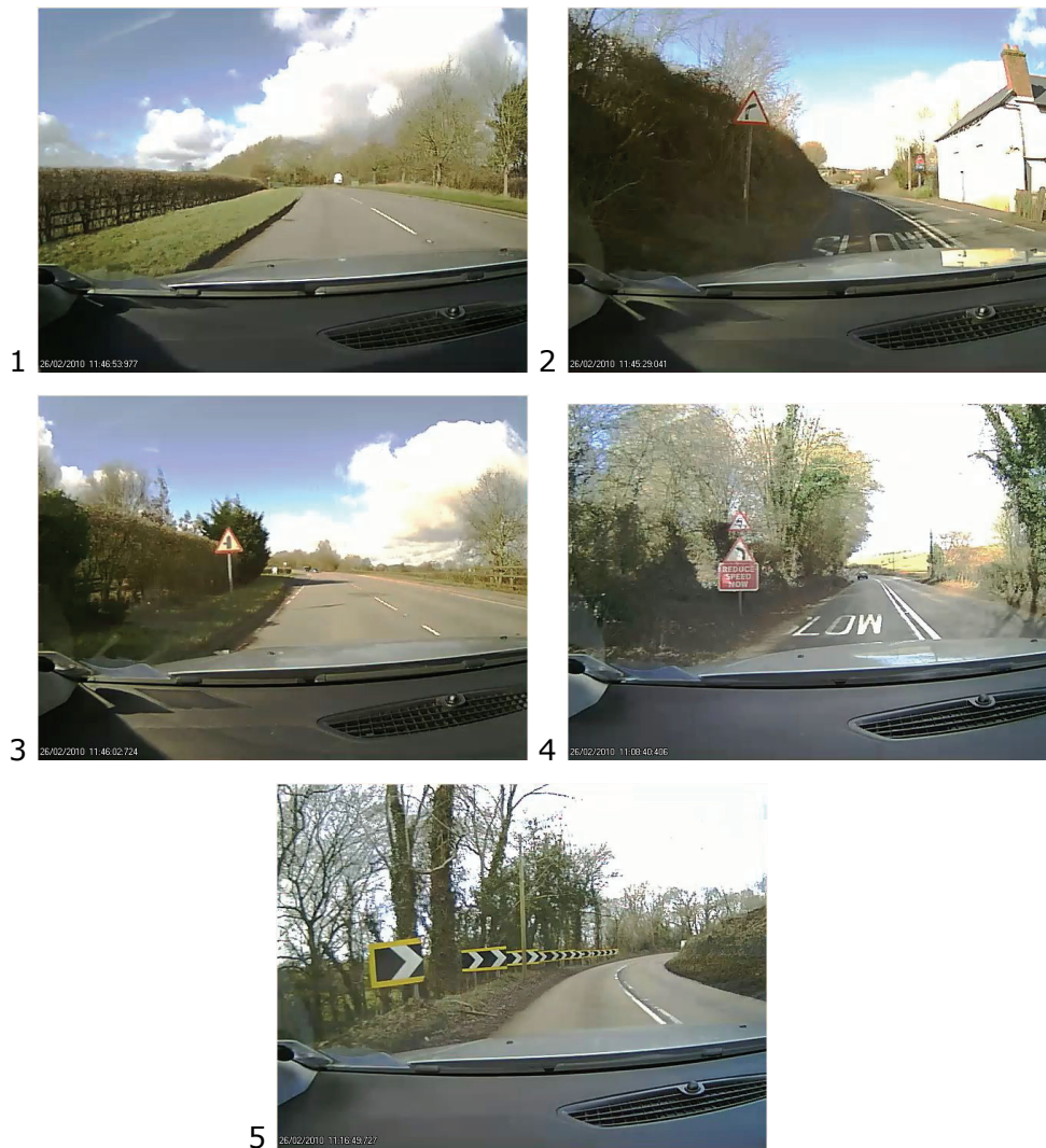
Figure 3-6: Examples of some of the different existing treatments associated with bends on the A377. These images are captured from the video footage of the drives.
