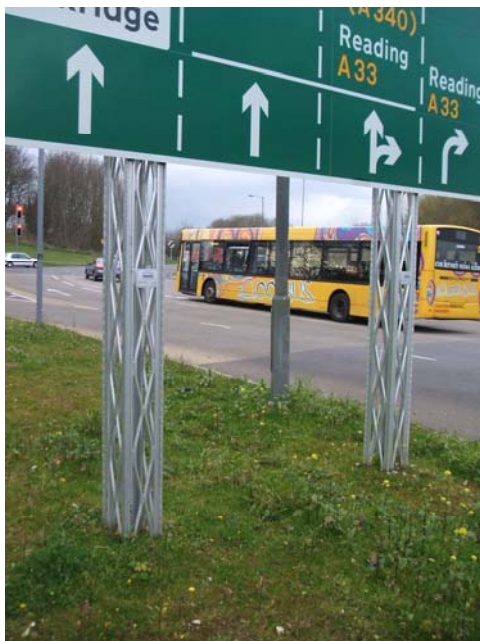
Figure 1: Passively safe signpost
