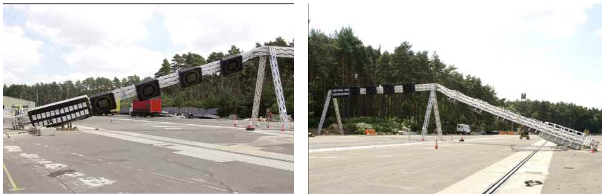
Figure 11: Gantry following collapse
