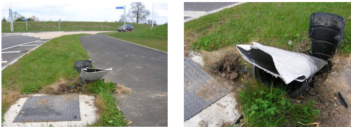
Figure 6: Category LE lighting column struck in Durham
