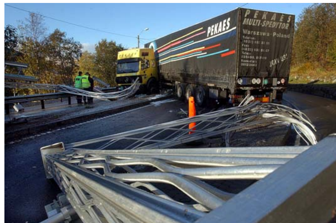
Figure 8: Collapsed gantry in Poland
