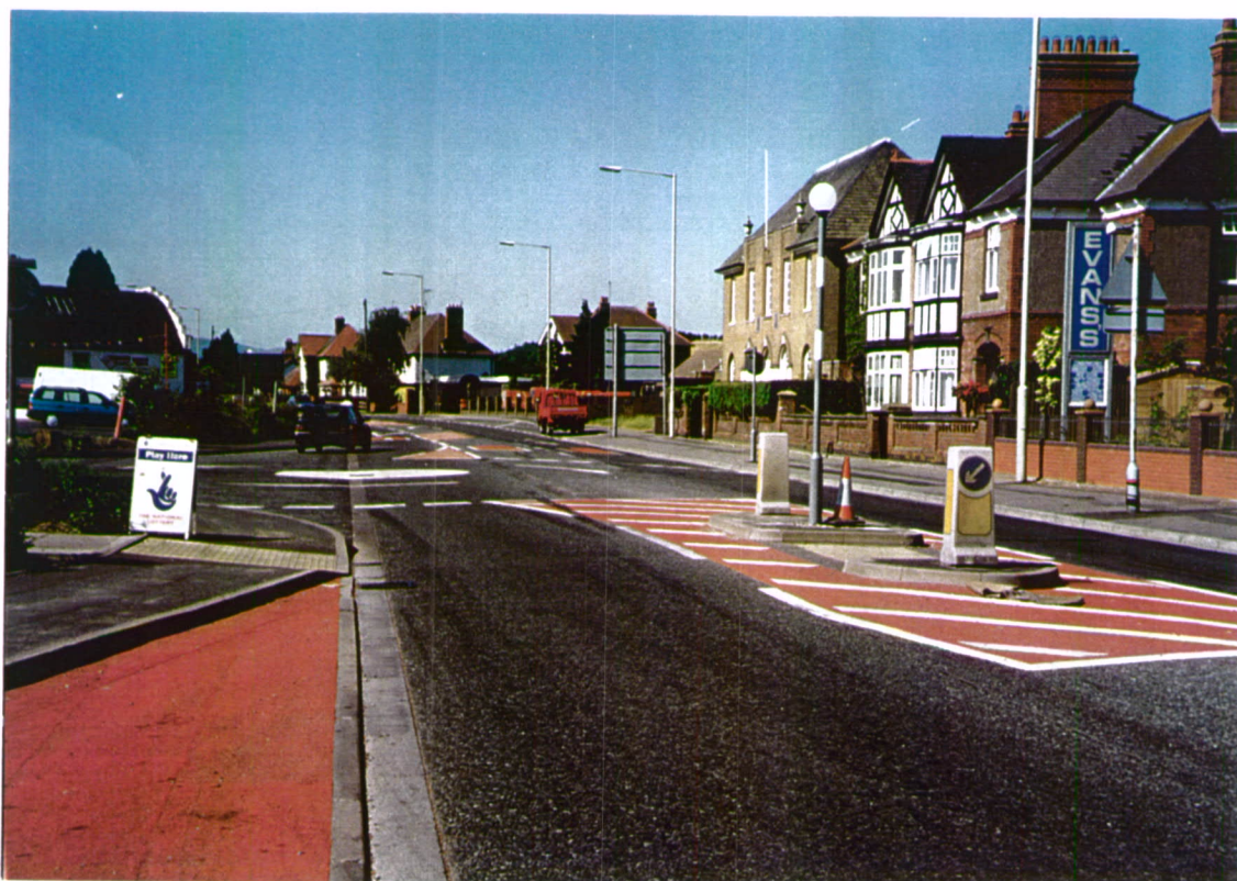
Fig 17. Mini-roundabout and pedestrian refuge outside the supermarket in the village centre, looking north (the refuge existed prior to scheme installation)
