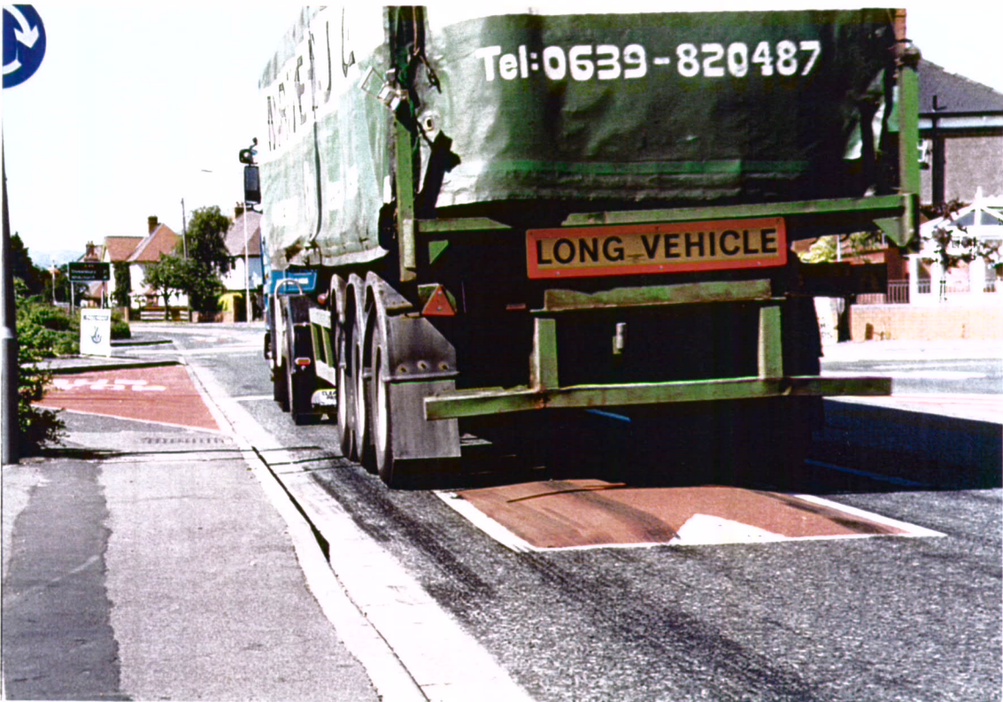
Fig 21. One of a pair of speed cushions on the northbound approach to the mini-roundabout junction with B4368 Corvedale Road, outside the supermarket (looking north)
