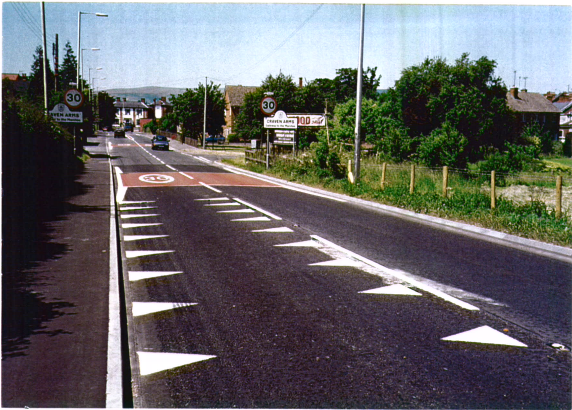
Fig 9. 'Dragon teeth' markings at the south gateway
