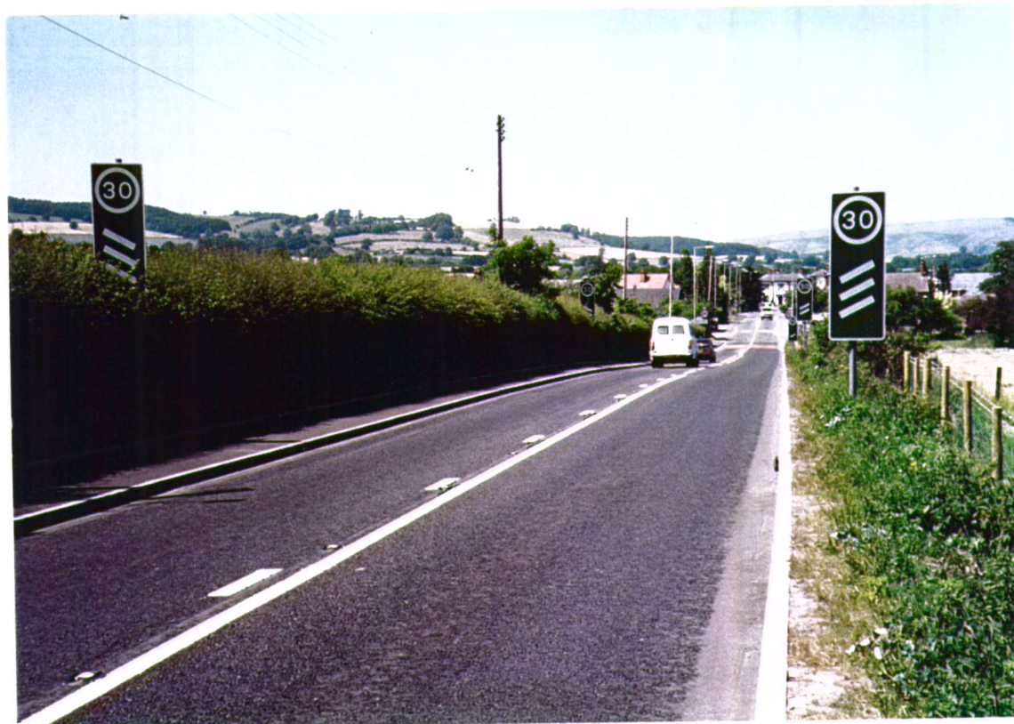
Fig 5. Countdown signs to the start of the 30mph speed limit at the south gateway (the pair illustrated are 150m from this speed limit)
