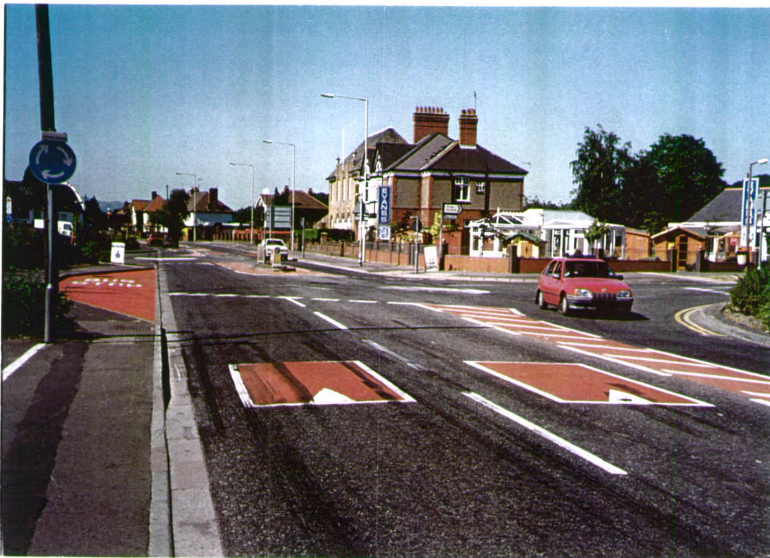
Fig 16. Speed cushions on the approach to the mini-roundabout at the junction with B4368 Corvedale Road, outside the supermarket in the village centre (looking north)
