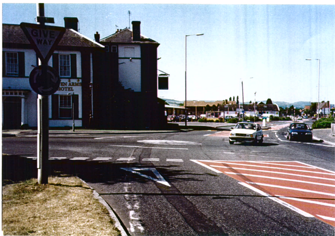
Fig 15. Mini-roundabout at the junction with the B4368 Clun Road, showing 'give way' signing and markings in addition to 'mini-roundabout' sign (looking north)
