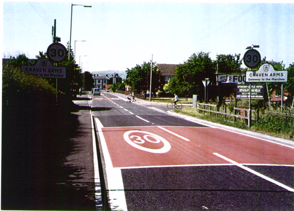
Fig 11. Textureflex surface treatment at the south gateway and associated markings and signing; the first repeated red patch with 30mph roundels can be seen in the distance
