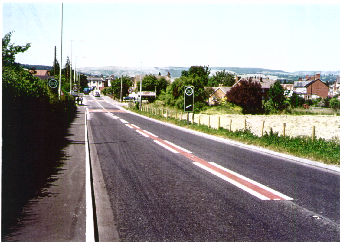
Fig 8. Red-infilled double centreline terminating 50m from the start of the 30mph speed limit at the south gateway - the 'dragon teeth' markings can be seen in the distance immediately in advance of the red surfacing at the gateway
