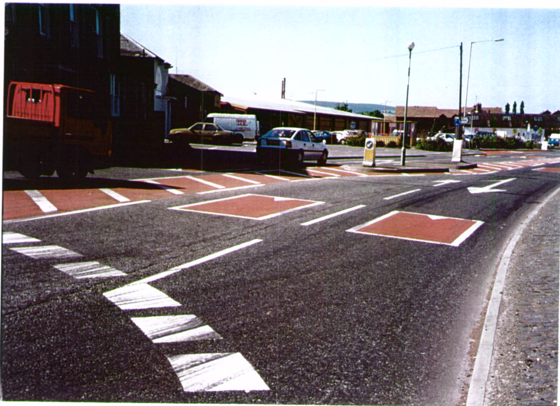
Fig 22. 'False speed cushions' (which are flat) on southbound approach to mini-roundabout junction with B4368 Clun Road, looking north (the refuge in the background existed prior to scheme installation)
