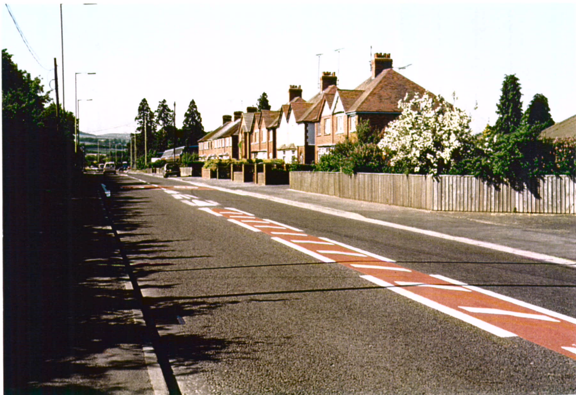
Fig 24. Centre hatching with red Textureflex infill in north of village (looking north); a repeated red patch is just visible in the distance
