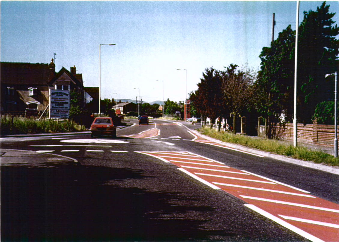
Fig 18. The northernmost mini-roundabout at the junction with White Meadow Close, showing nearside hatched deflection for oncoming traffic (looking north)
