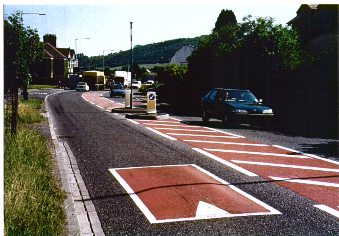
Fig 19. Speed cushion, pedestrian refuge and centre hatching just north of village centre (looking south); another cushion is just visible beyond refuge in opposite lane
