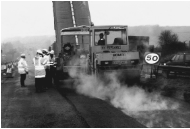
Figure 2 Laying and compaction in cold weather at Site C
