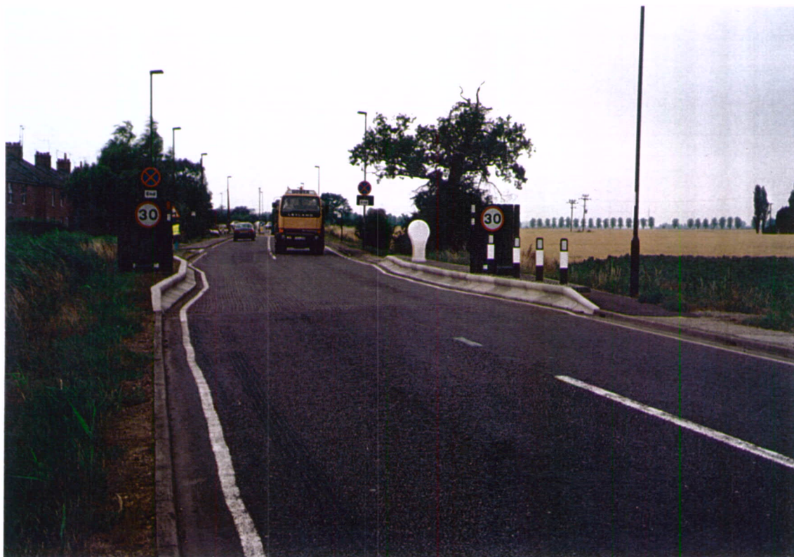
Fig.7 East gateway, showing narrowing with Trief kerbing, speed limit roundels fixed to Chevrolflex plastic strips and Imprint surface treatment
