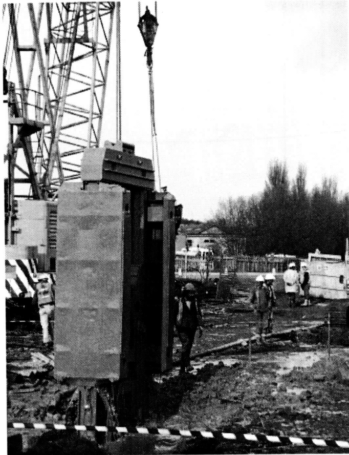
(a) Panel excavation
