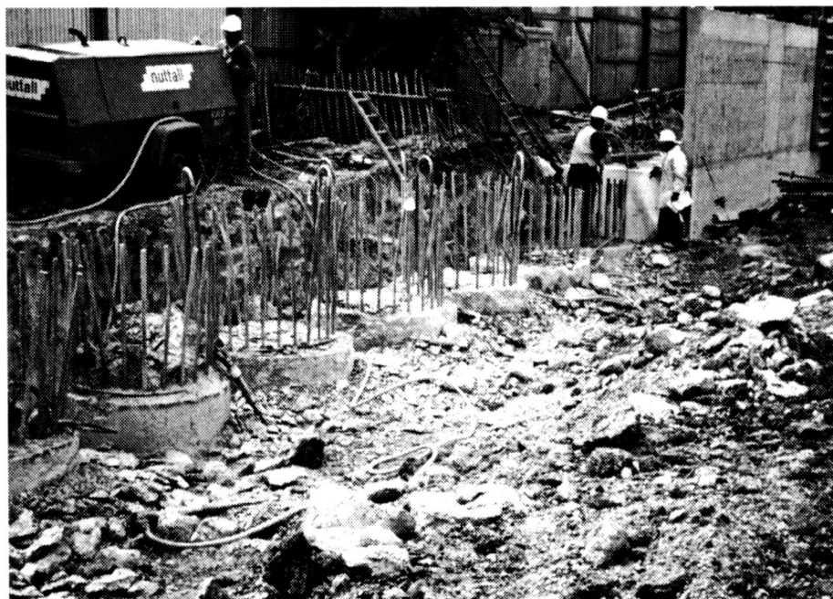
Fig 6. Pile tops being trimmed to cut-off level
