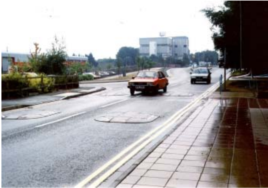
Plate 6 Vehicle manoeuvring centrally between speed cushions — Billing Brook Road (site 25) (Picture courtesy of Northamptonshire CC)
