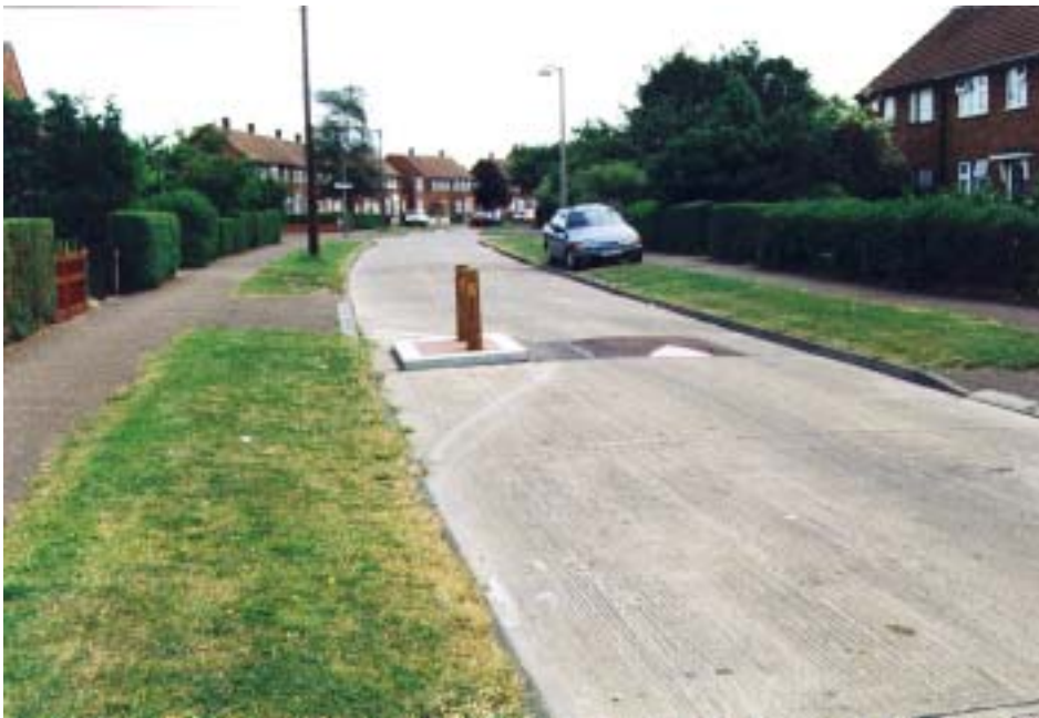
(b) Single cushion layout - single buildout — Chapelfields Area (site 15) (Picture TRL)
