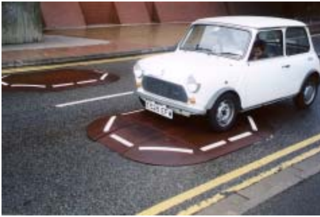
(a) Moulded rubber cushions Billing Brook Road (site 25) (Picture courtesy of Northamptonshire CC)
