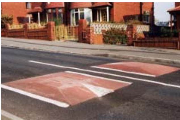
(e) Pre-formed concrete cushions Chadderton Park Road (site 9) (Picture courtesy of Oldham MBC)
