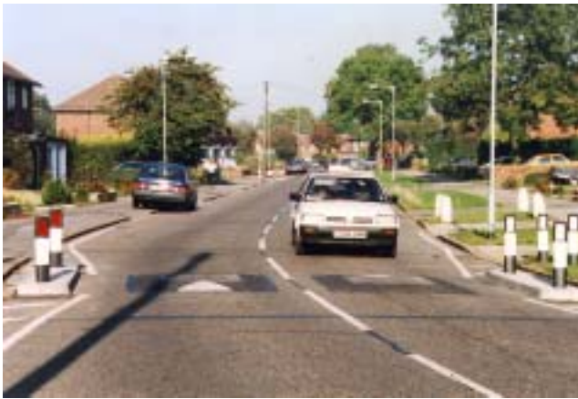
(c) Cushion pair within pinch point Windmill Road (site 8) (Picture courtesy of Hertfordshire CC)
