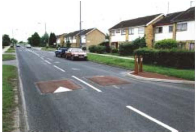
(d) Cushion pair at single buildout Foxwood Lane (site 19) (Picture TRL)
