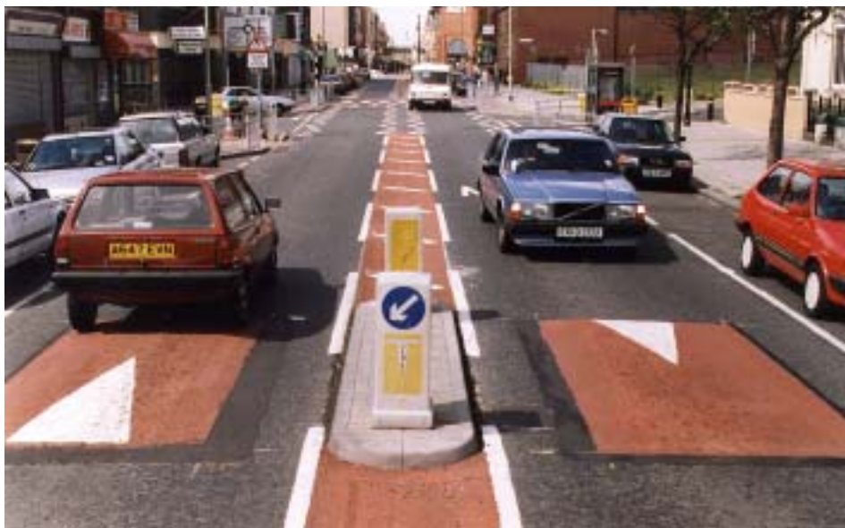
(b) A183, local distributor road with asphalt cushions — Ocean Road (site 29) (Picture courtesy of South Tyneside MBC)
