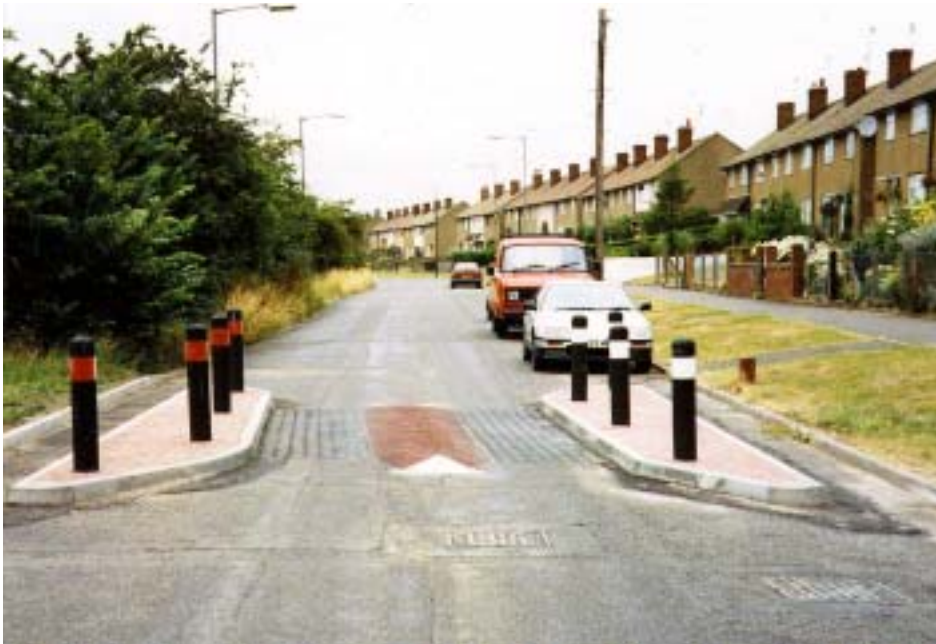
Plate 9 Long narrow angled cushion within a chicane — Camp Hill (site 30) (Picture courtesy of Warwickshire CC)
