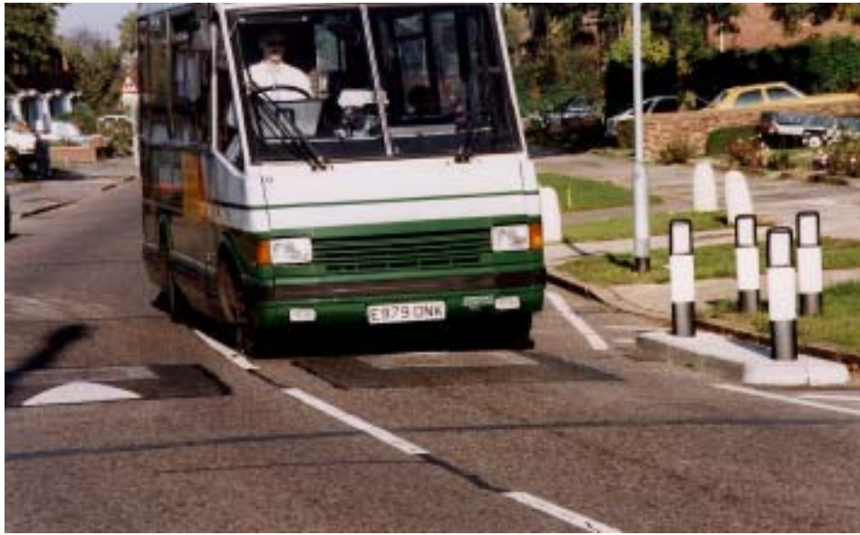
(a) Midibus approaching cushions — Windmill Road (site 8) (Picture courtesy of Hertfordshire CC)
