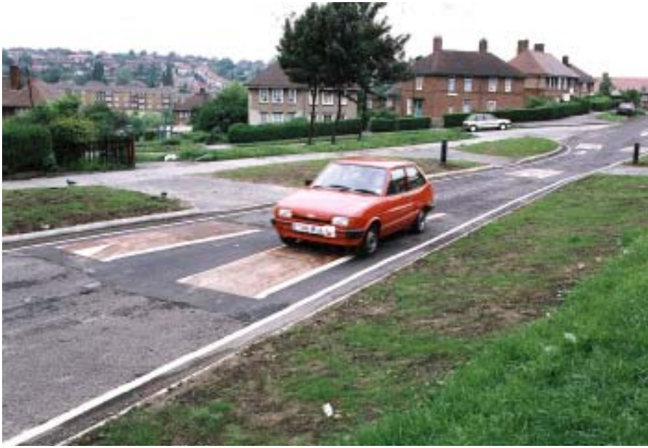
Plate 8 Vehicle crossing a group of 5 cushions at a pinch point — Lindsay Avenue (site 28) (Picture TRL)
