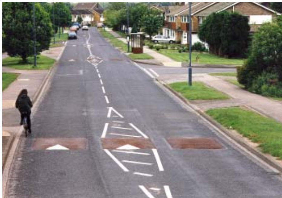
Plate 7 Three-abreast cushion layout — Foxwood Lane (site 19) (Picture TRL)
