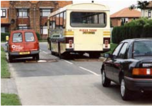
(a) Cushion pair without buildouts or islands Muncaster (site 22) (Picture TRL)
