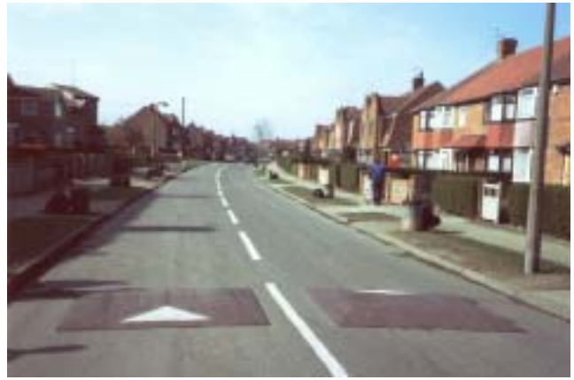
(b) Moulded rubber cushions Muncaster (site 22) (Picture TRL)
