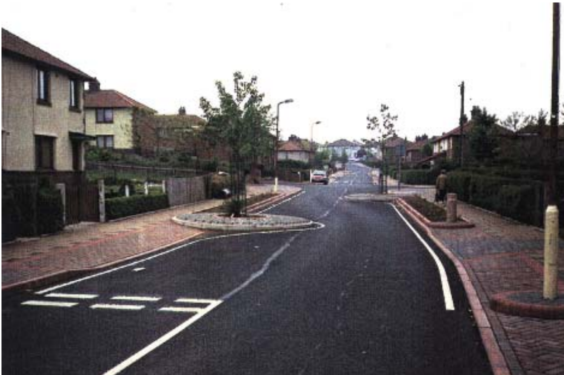
Plate 10 Example of a chicane incorporating planters: Scheme 8, Dalton Avenue
