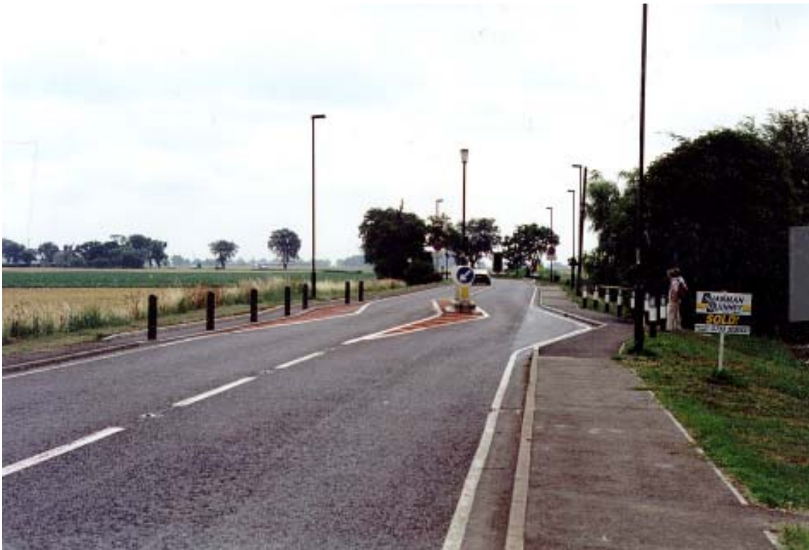
Plate 4 Example of a two-way working chicane: Scheme 36, A47 Thorney
