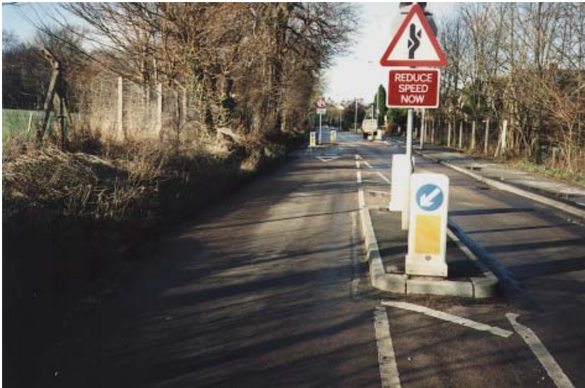
Plate 7 Sign warning of a chicane ahead, with supplementary ‘reduce speed now’ plate, at Scheme 20, Bushey Mill Lane
