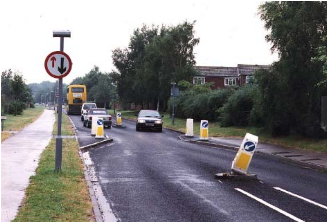
Plate 9 Damage to a bollard at a chicane, Great Hollands, Bracknell
