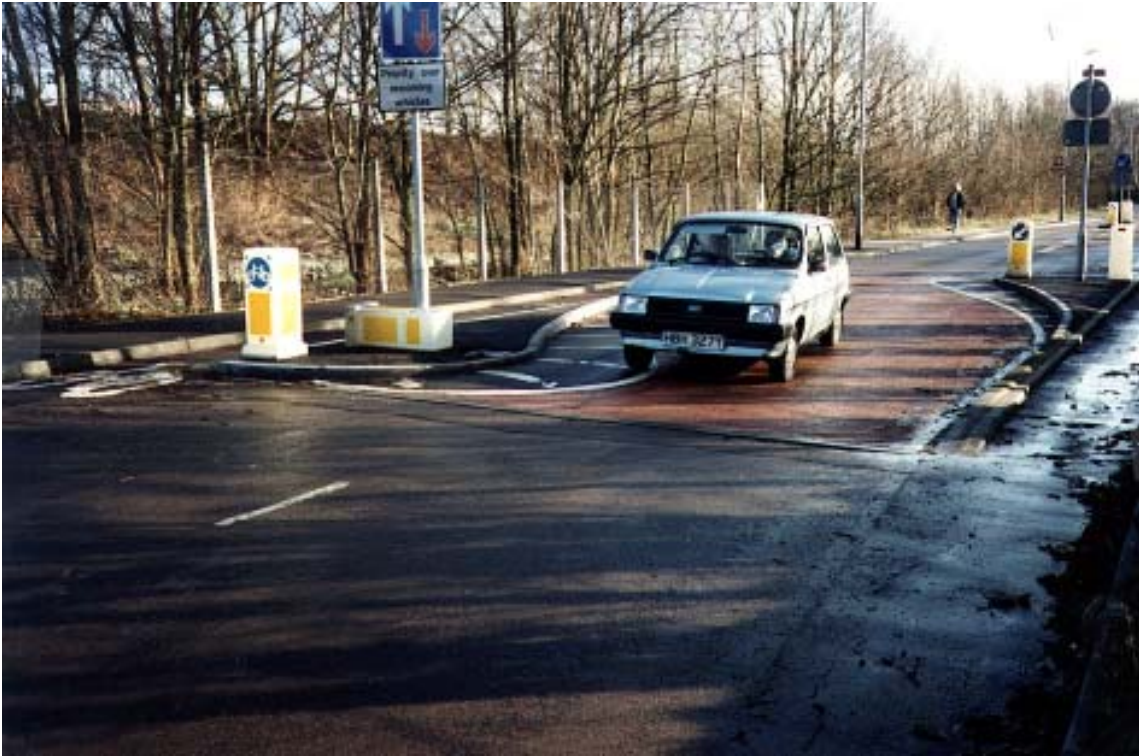
Plate 5 Example of a single lane working chicane with overrun areas: Scheme 20, Bushey Mill Lane
