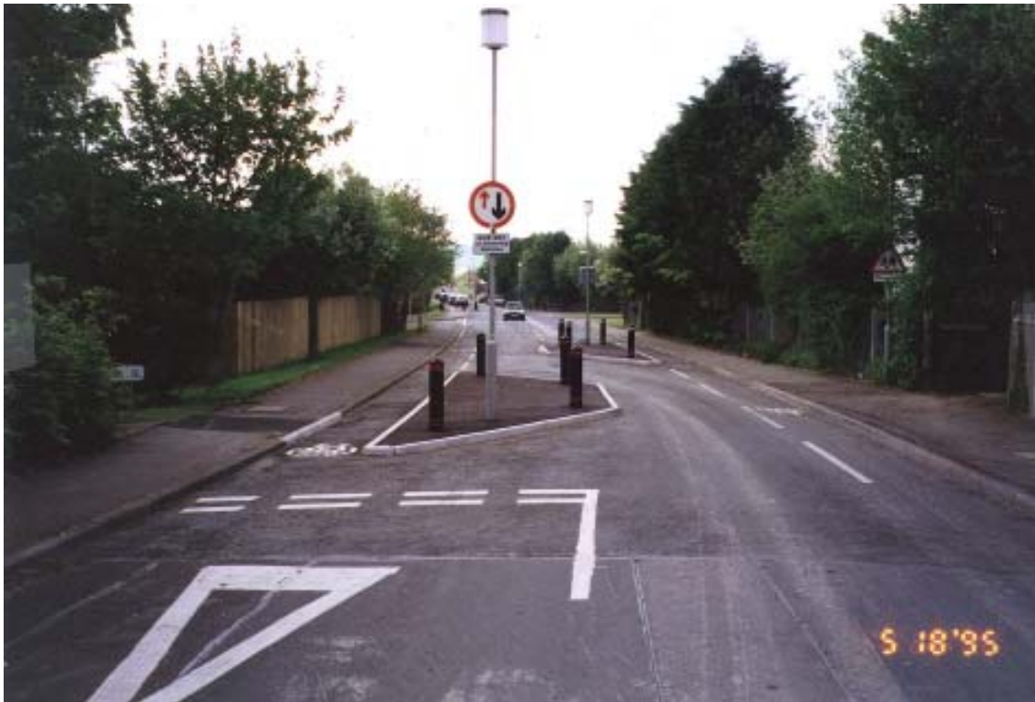
Plate 1 Example of a single lane working chicane with cycle lane bypass: Scheme 9, Maiden Castle Road
