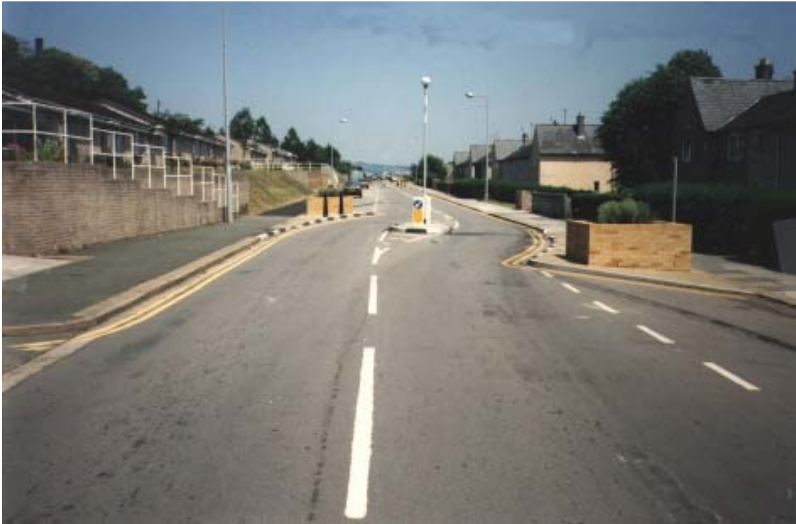
Plate 3 Example of a two-way working chicane: Scheme 37, Beaumont Road
