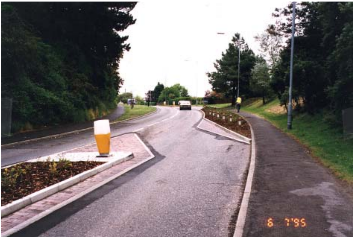
Plate 6 Example of a two-way working chicane with overrun areas: Scheme 46, A149 Cromer
