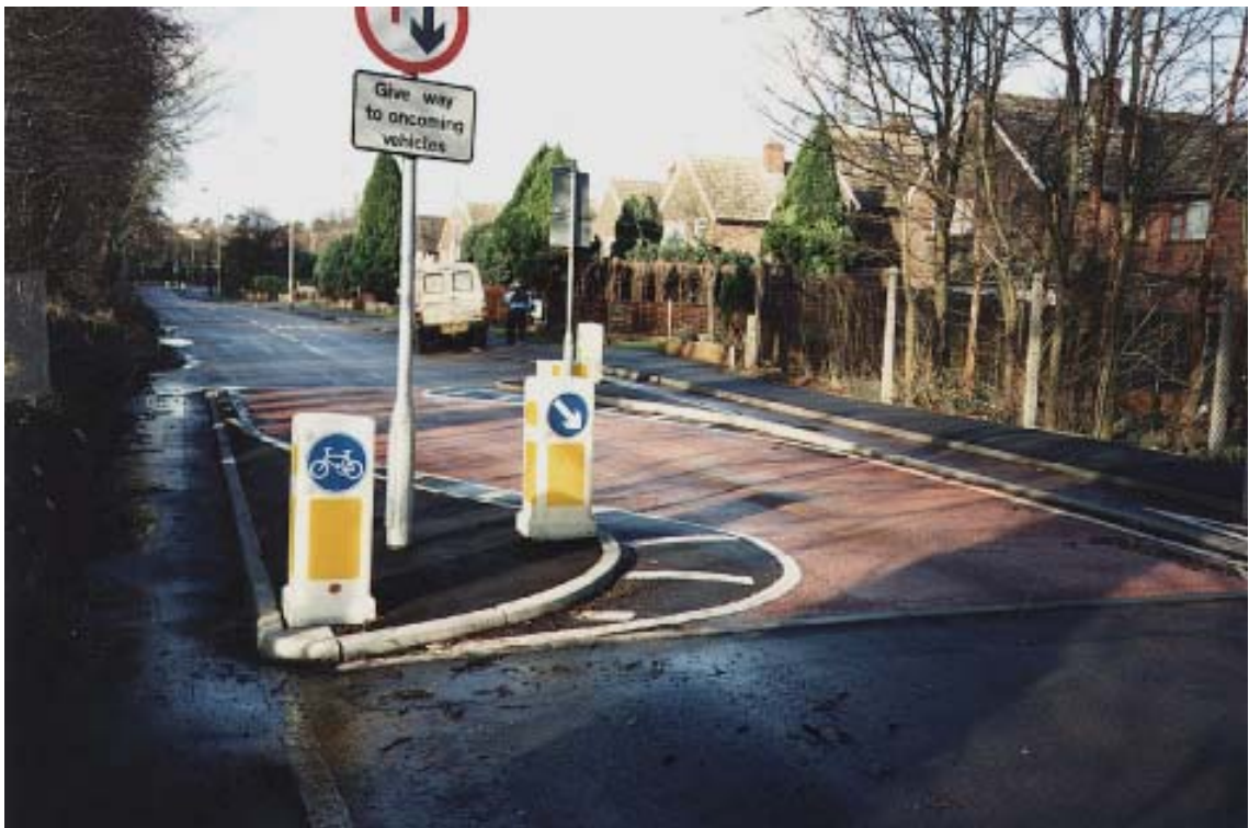
Plate 8 Example of signing at a single lane working chicane with cycle bypass: Scheme 20, Bushey Mill Lane
