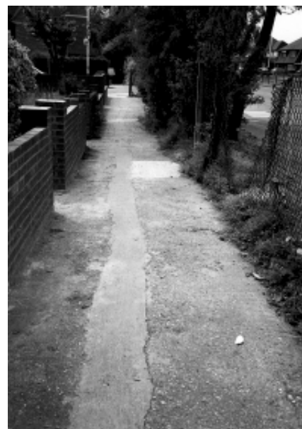
Plate 21 Good quality concrete reinstatement
