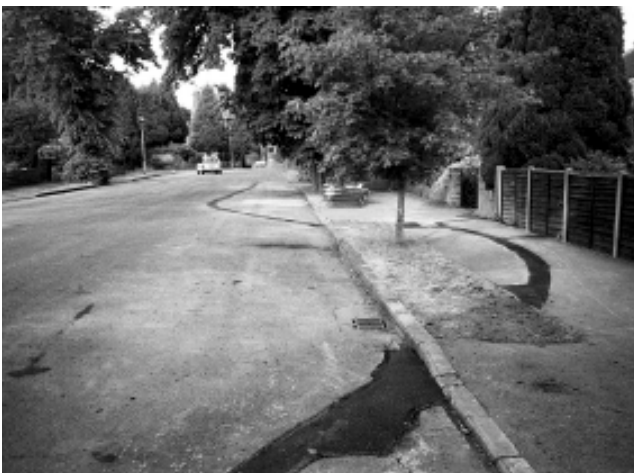
Plate 18 Avoiding tree roots (poor planning)
