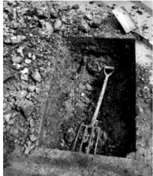
Plate 8 Good quality saw cut opening
