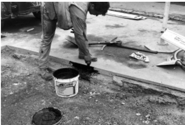
Plate 11 Use of edge-sealing material
