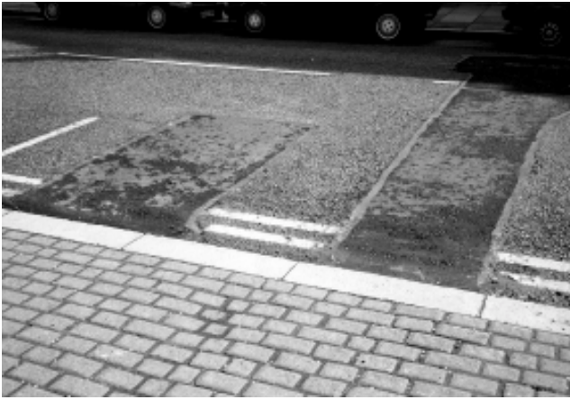
Plate 22 Good quality carriageway reinstatement
