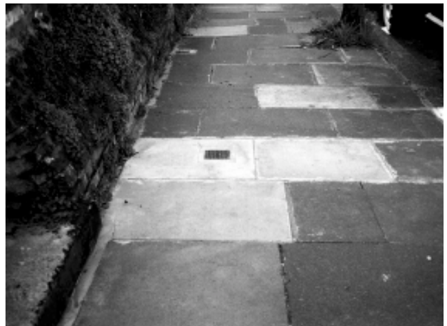
Plate 20 Good quality modular reinstatement
