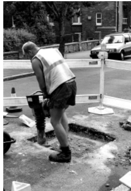
Plate 9 Correct compaction procedure
