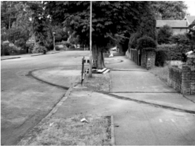
Plate 17 Avoiding damage to tree roots (poor planning)
