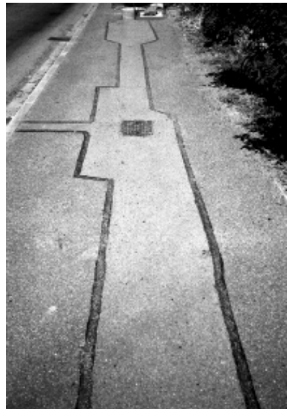
Plate 19 Good quality flexible reinstatement
