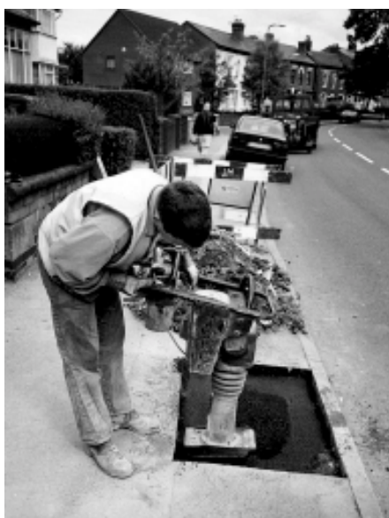
Plate 13 Good compaction technique (bound materials)
