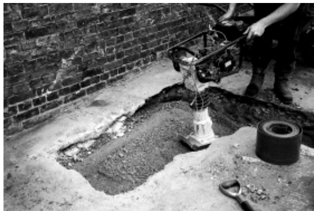
Plate 14 Good compaction technique (unbound materials)
