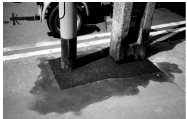
Plate 10 Good quality permanent reinstatement
