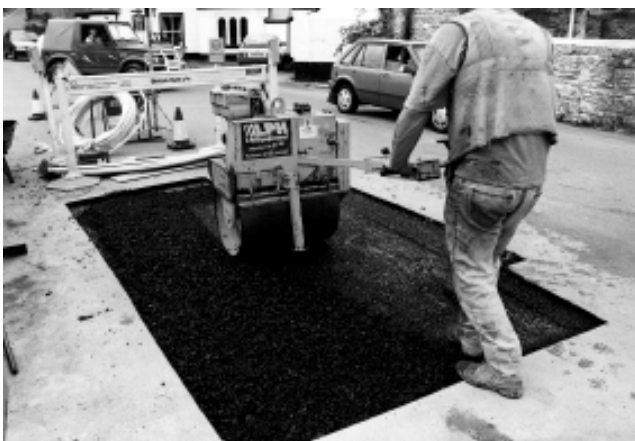
Plate 12 Good compaction technique (bound materials)
