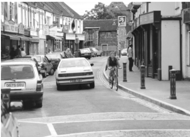
Plate 6 Contra-flow scheme in St Marks Road, Bristol looking south
