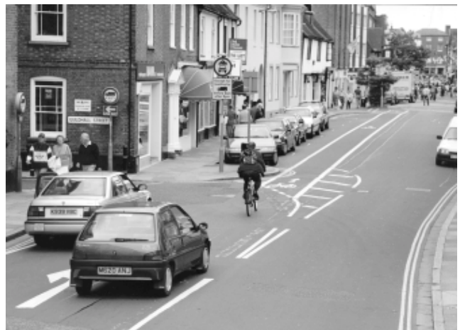
Plate 7 Entrance to contra-flow scheme in North Street, Chichester
