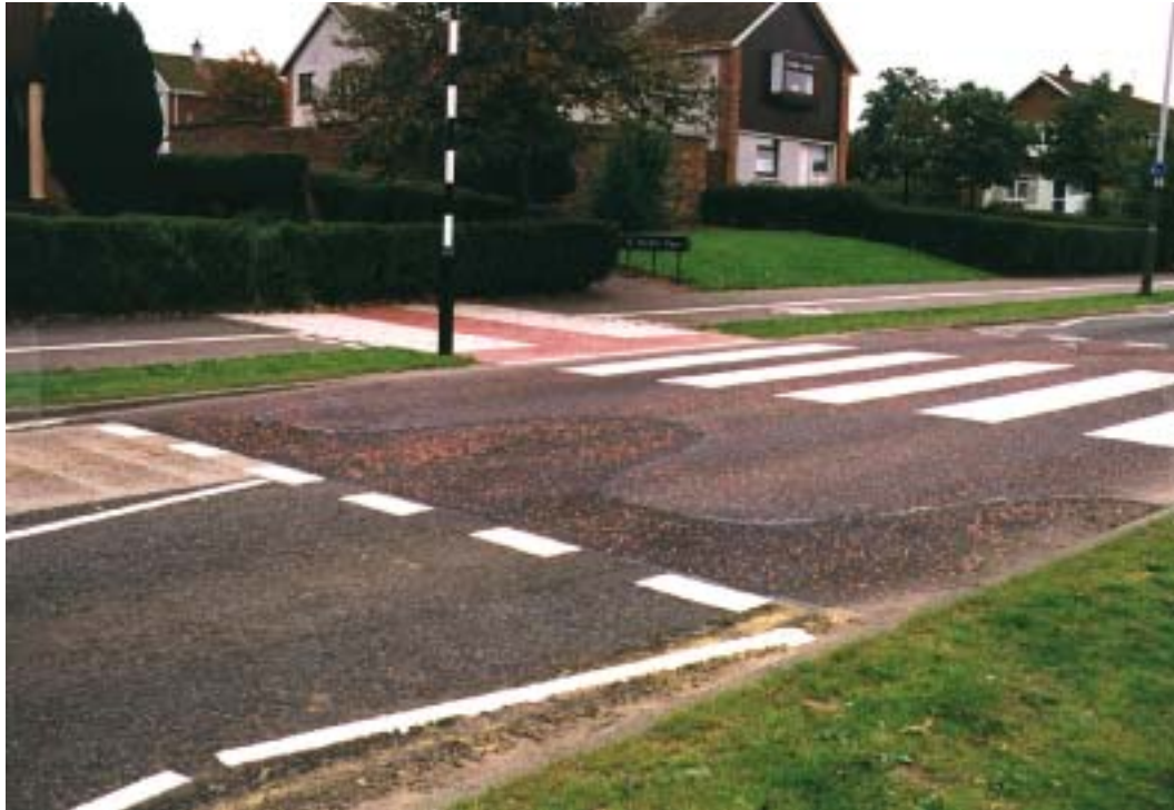
Figure 12 'S' hump at a raised zebra crossing on South Parks Road, Glenrothes
