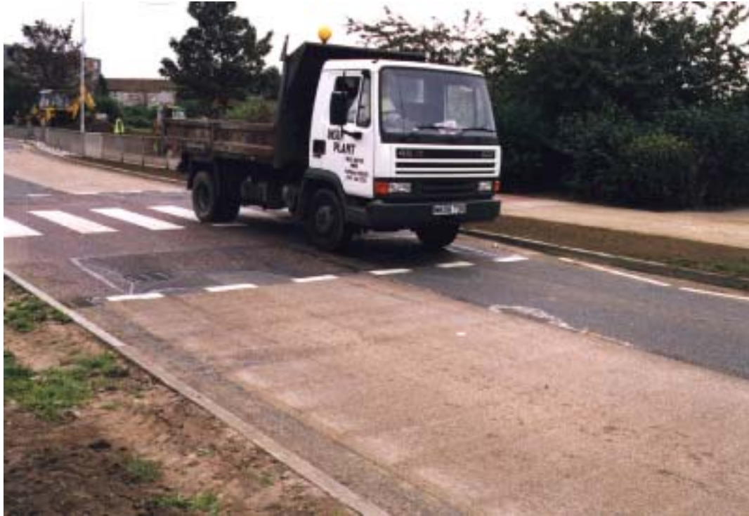
Figure 10 'H' hump at a raised zebra crossing on South Parks Road, Glenrothes
