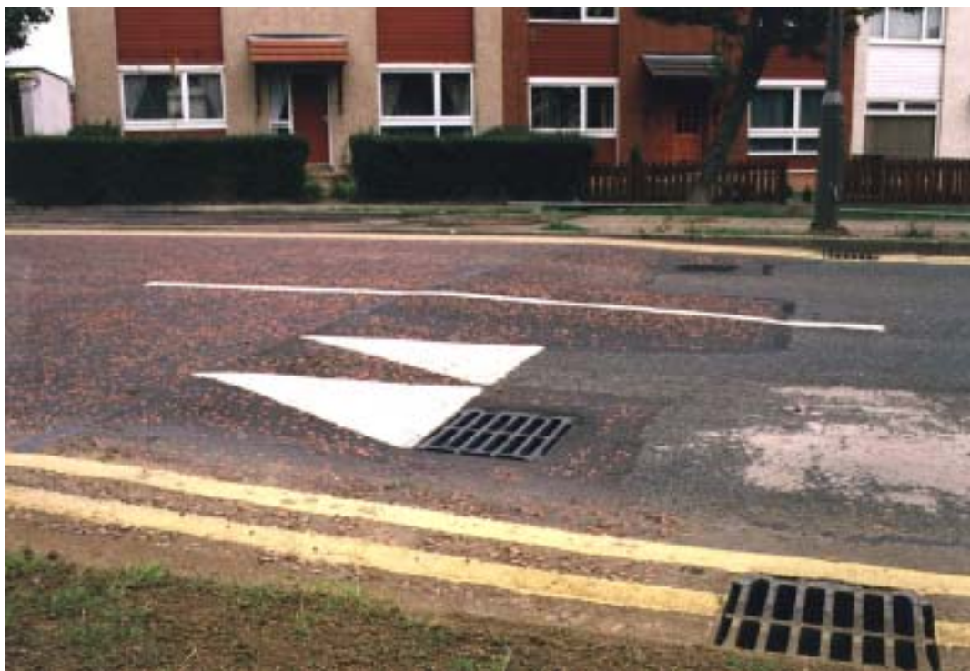
Figure 11 'H' hump ramps and drainage gullies on South Parks Road, Glenrothes
