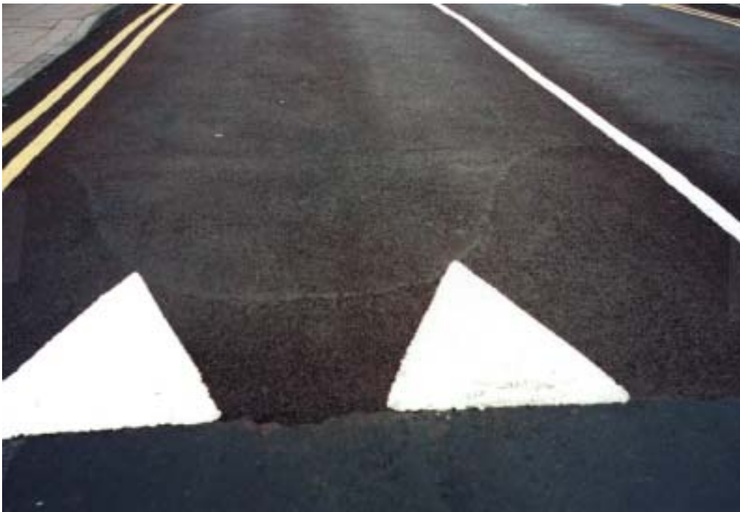
Figure 15 'S' hump at Northampton showing the continuous curve between bus and car ramps
