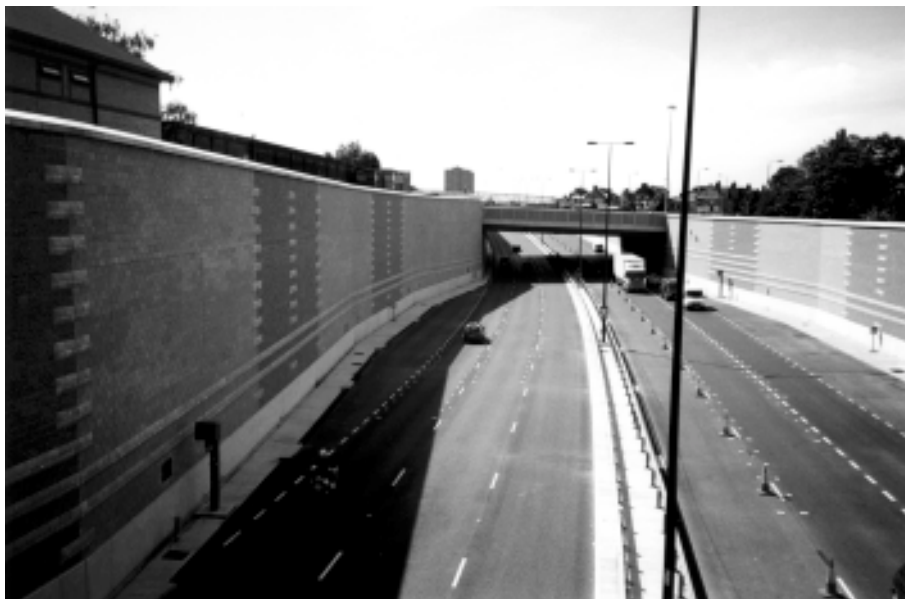
Plate 1 The completed wall at chainage 3540
