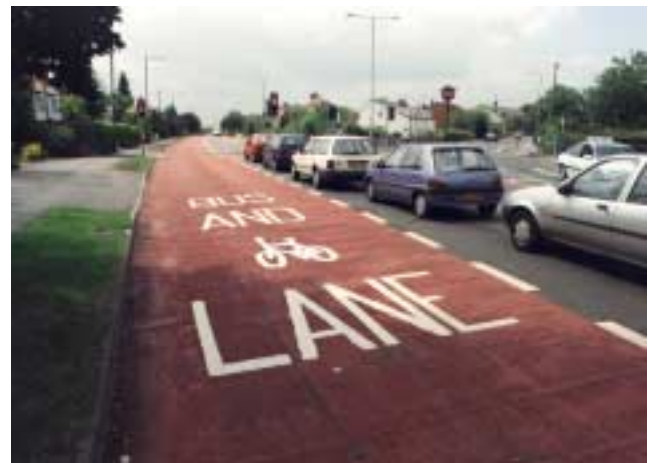
Figure 5 Bus and cycle lane, Cheltenham Road (1997-98)
