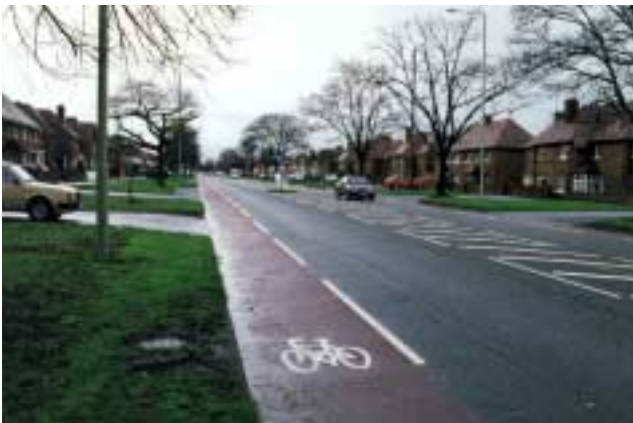
Figure 3 Carriageway narrowing (central hatching and refuges) and cycle lane, Finlay road (1996-97)
