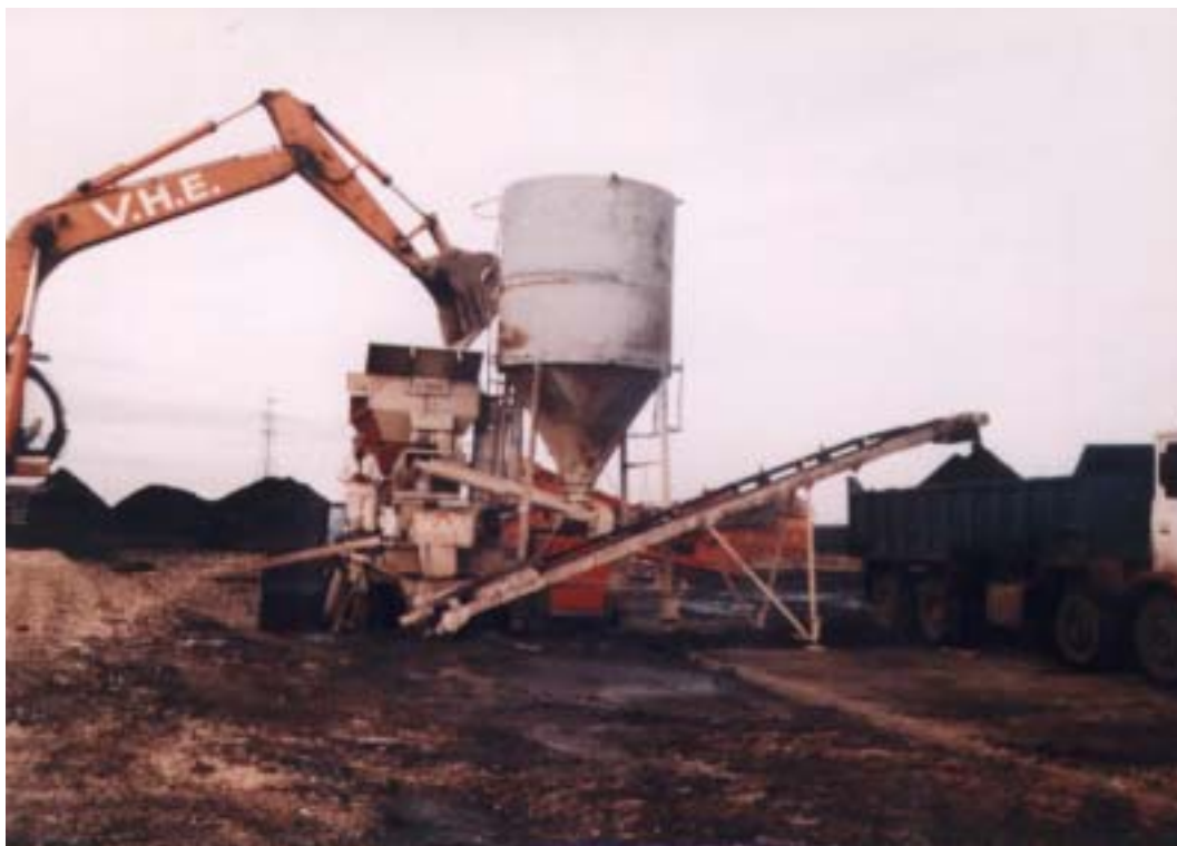
Plate 1 Belmix batching plant used for S/S treatment
