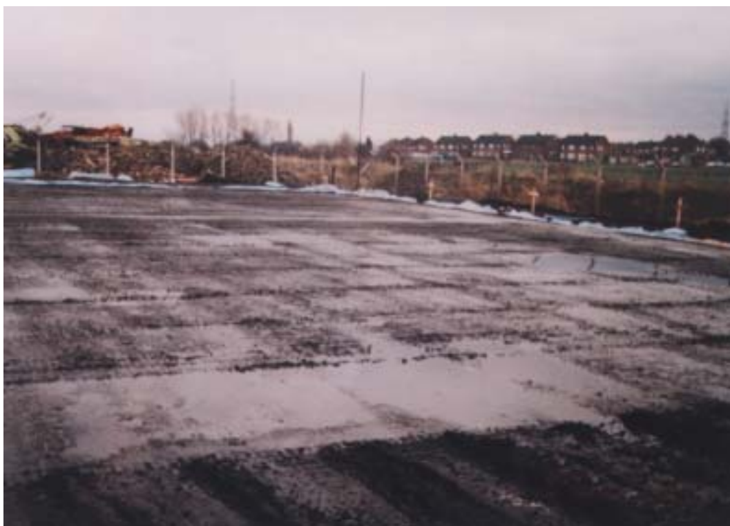
Plate 2 Construction of main slab December 1994
