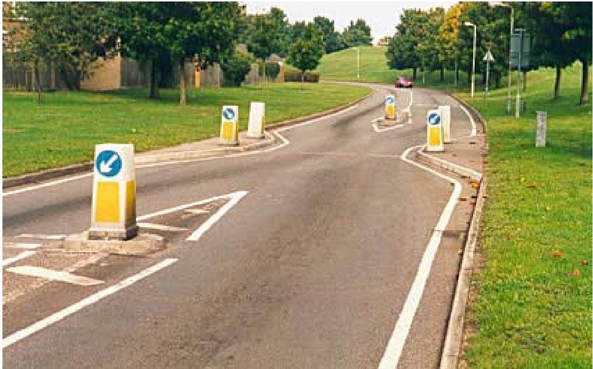
Figure 15 Chicane: Great Hollands Road, Bracknell
