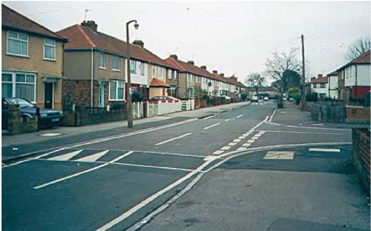
Figure 13 Raised junction: Carlton Road, Slough
