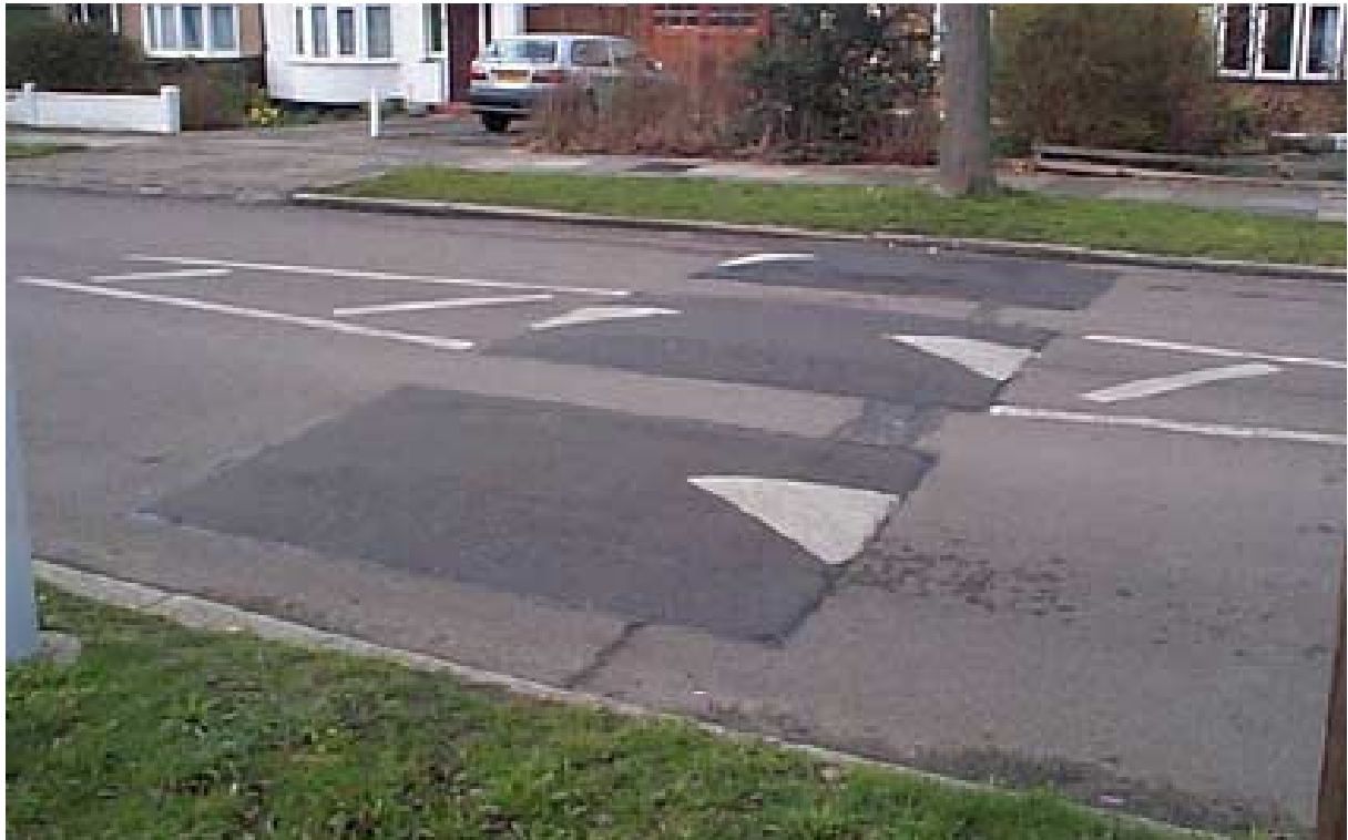
Figure 9 1.7m-wide speed cushions: Welbeck Road, Harrow
