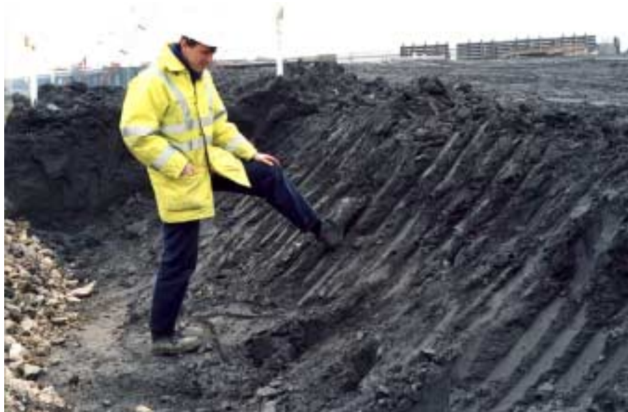
Plate 2 Lime modified silt in-situ nine months after construction
