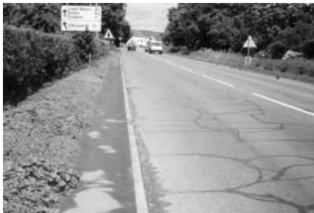
Figure 1 Overbanding on A38 Edithmeade to Cross (Chart 1140)
