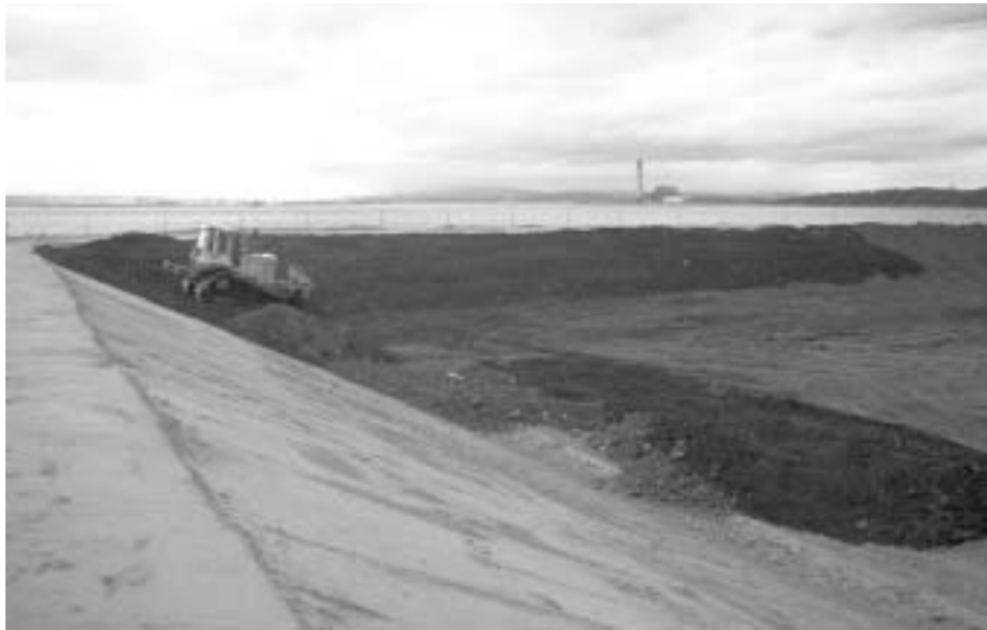
Figure 10 Construction of a pulverised-fuel ash disposal lagoon dam. Note that the sideslopes are in the process of being covered to provide protection from the weather
