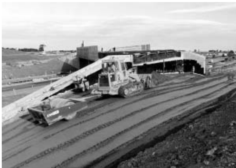
Figure 14 Pulverised-fuel ash compaction during construction of the M1–A42 Link
