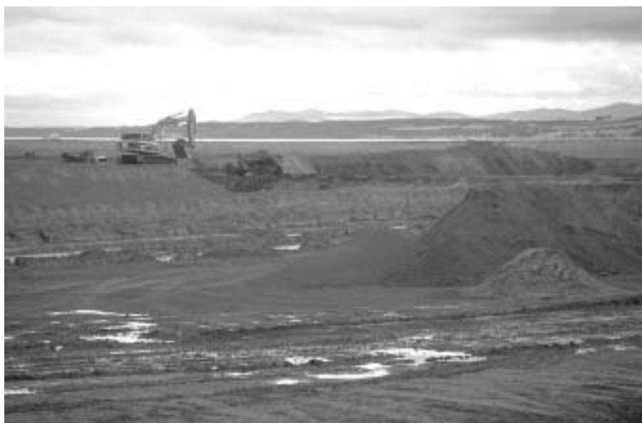
Figure 1 A typical pulverised-fuel ash disposal lagoon at the time of excavation
