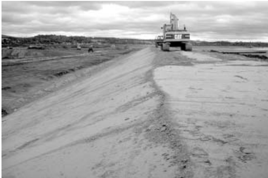
Figure 4 Construction of a pulverised-fuel ash disposal lagoon dam
