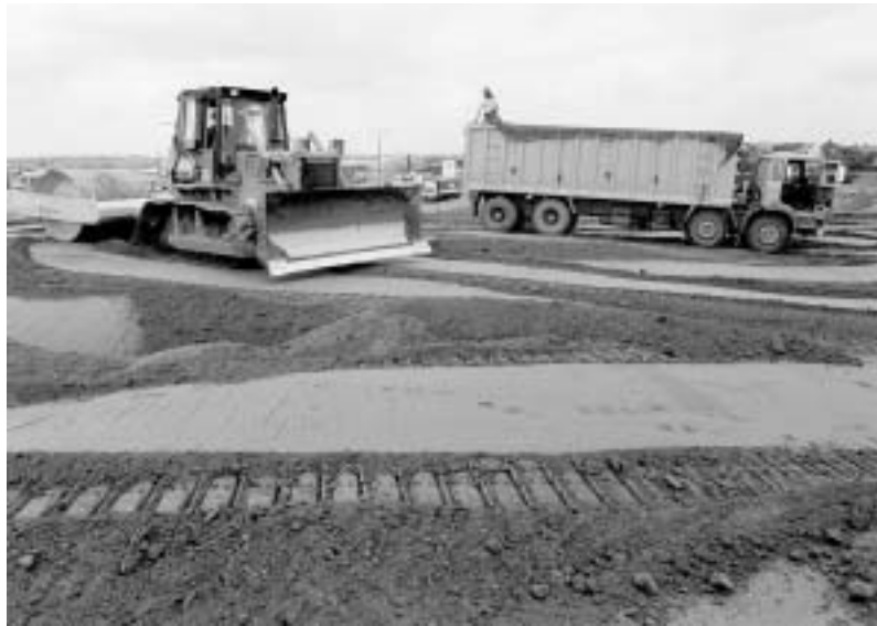
Figure 12 Pulverised-fuel ash compaction during construction of the A52 trunk road
