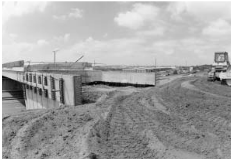
Figure 13 Pulverised-fuel ash compaction during construction of a new flyover approach road on the A52 trunk road
