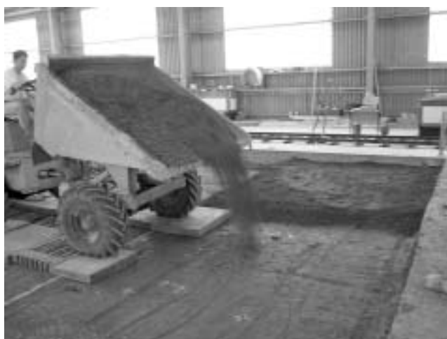
Figure 8 Delivery of materials
