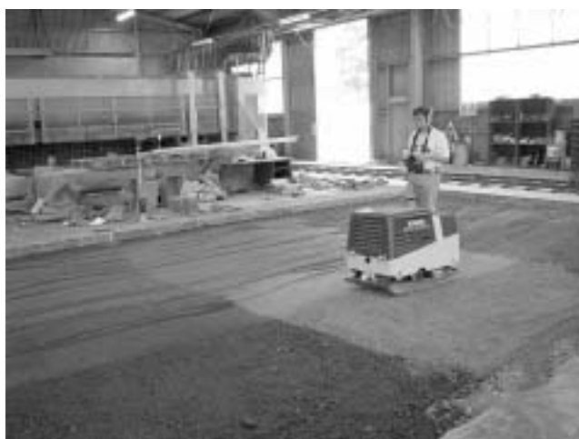
Figure 9 Compaction of four bays
