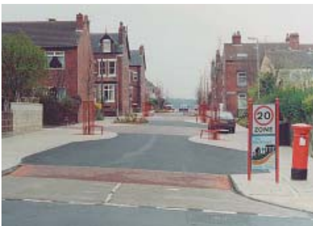
Figure 3.2 Gateway at western end of Methley Drive
