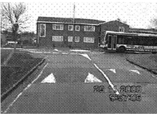
Road hump/mini roundabout – Links 16/17
