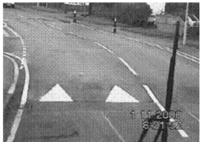
Road hump – Link 18a
