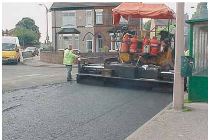
Figure A1 Utilisation of crushed glass as a aggregate in road construction
