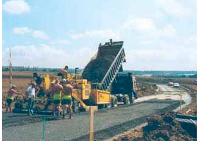
Figure A4 Application of IBA in CBM, Waltham Abbey (Ballast Phoenix)
