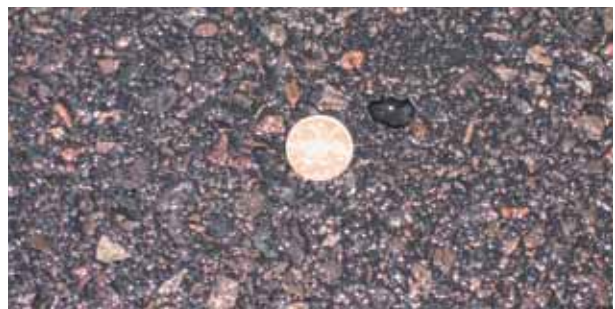
Figure 3.9 Treated surface – after water jetting (Site TSMA8)
