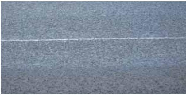
Figure 3.10 Good joint at Site TSMA12 (ten years)
