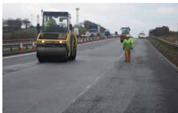
Figure 7.2 Newly-laid surfaces – 0/14 mm SMA (background) and 0/10 mm SMA (foreground)
