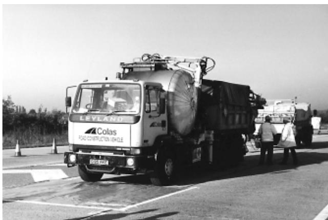
**Figure 1** Laying equipment for acrylic-resin system
