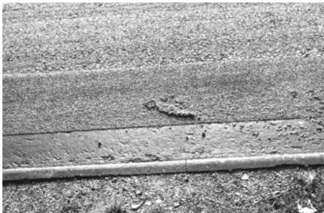
**Figure 2** Underlying material showing through acrylic-resin system
